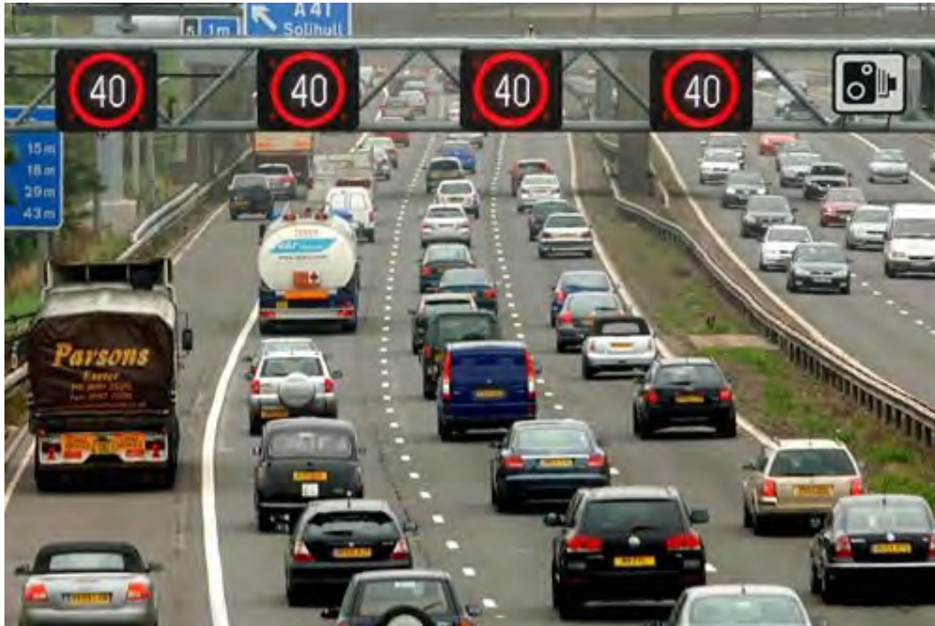
Figure 4.3: Variable Speed Advisory on Multiple Lanes. (The Red Circle Around the Speed Limit Denotes whether the Speed Limit is Advised or Enforced.)
