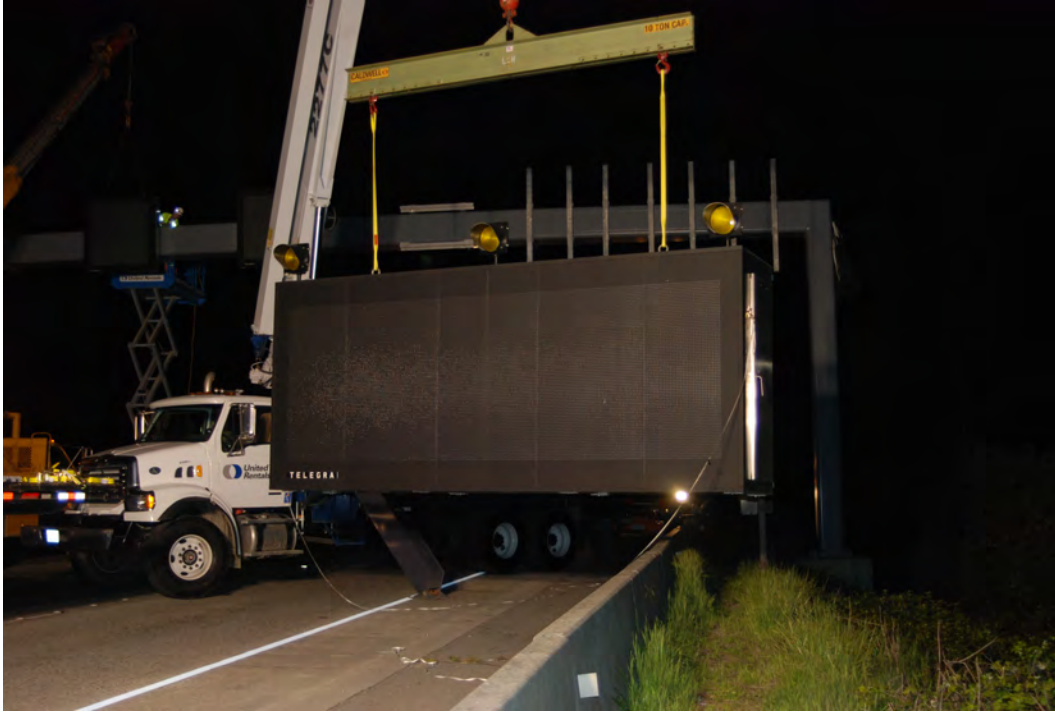
Figure 4.2: Installation of Variable Message Sign Requires Heavy Equipment
