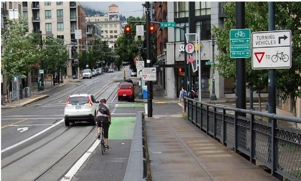
Figure 13 Quadrupole inductive loop in bike lane at NW Lovejoy and 9th Ave.
