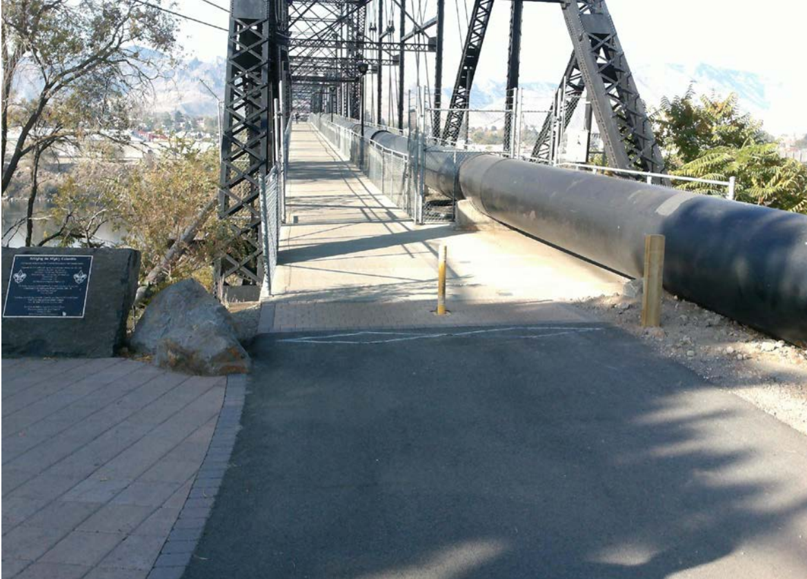
Figure 12 Apple Capitol Loop Trail, Old Wenatchee Bridge.
