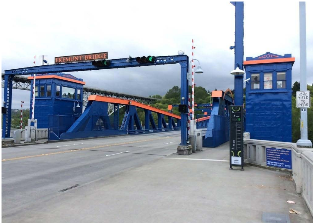
Figure 11 Fremont Bridge Eco-Totem
