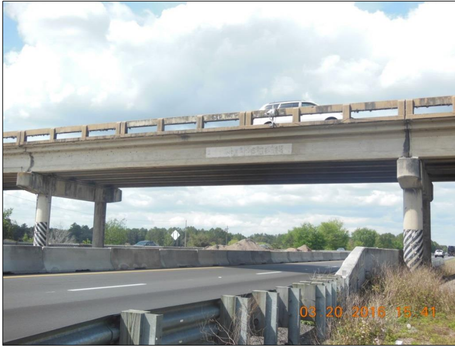
Figure B-0-3: Bracket on Overpass at Location 3
