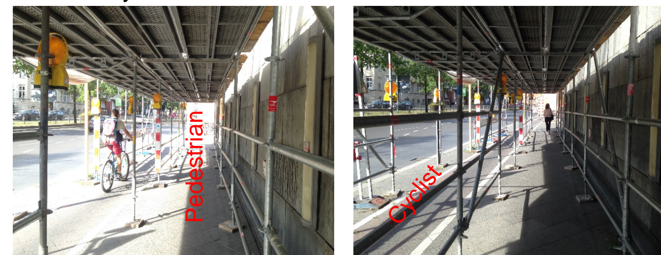
Figure 3: Covered pathways for cyclists and pedestrians
