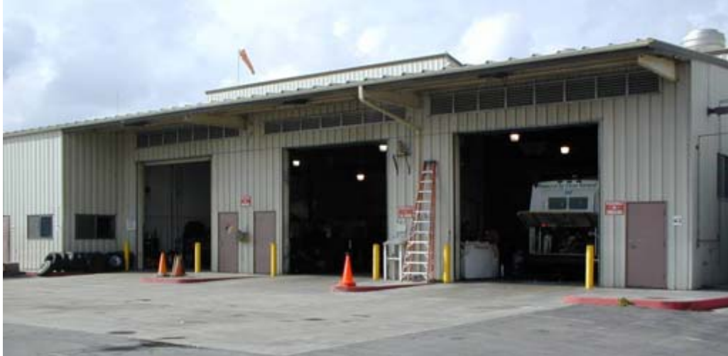
Figure 17. CNG maintenance facility in Thousand Palms
