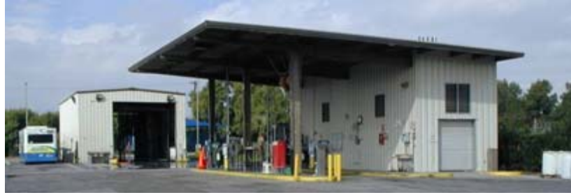
Figure 8. CNG fueling lane and bus wash (Thousand Palms)
