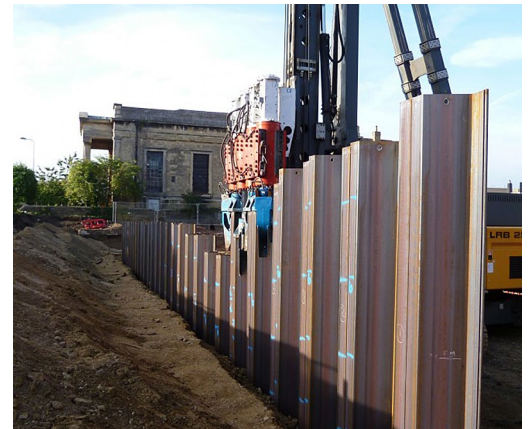
Installation of a sheet wall pile.
