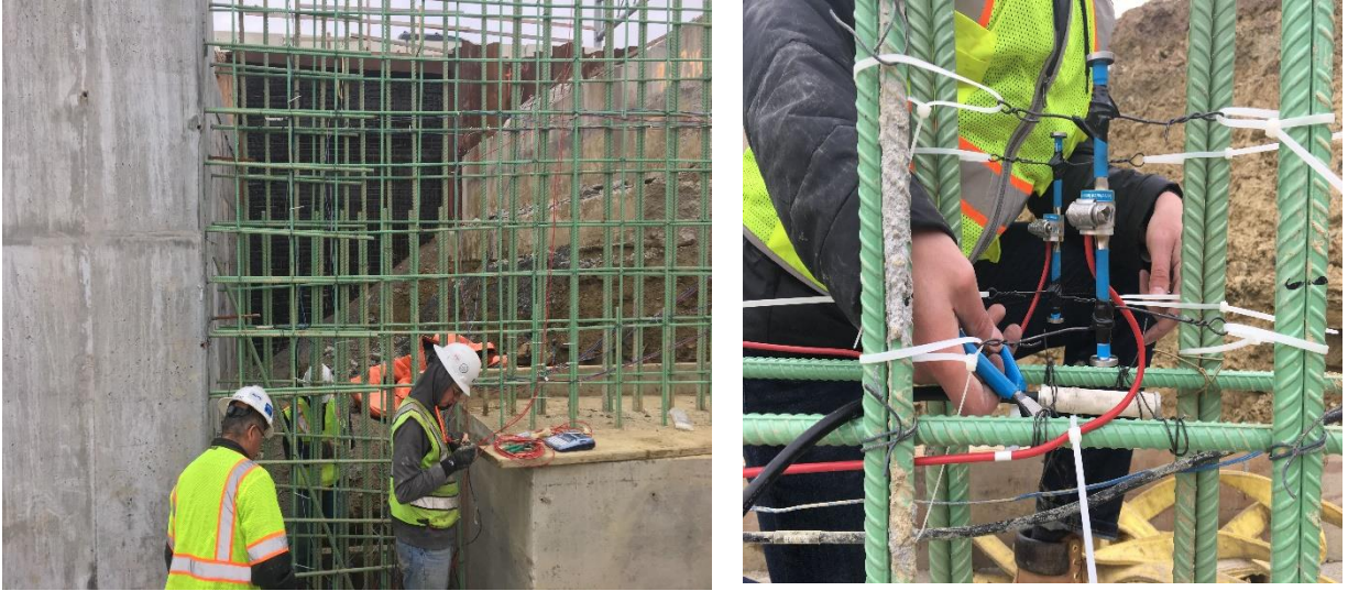
Figure 12. Installing strain gages in the wingwall.
