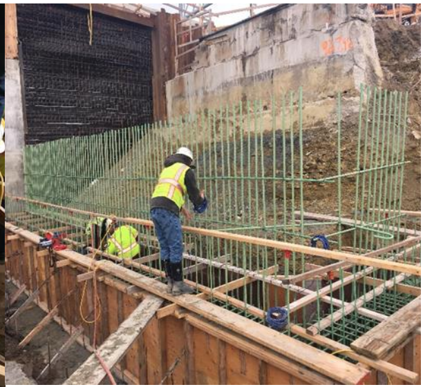
Figure 11. Installing strain gages in the footing.
