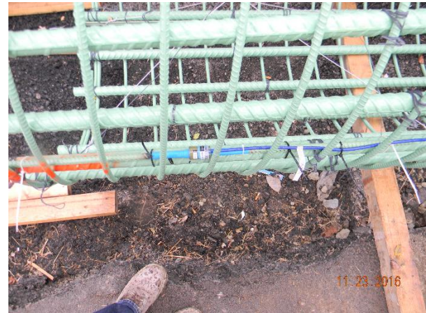
Figure 10. Installing strain gages in the drilled shafts.
