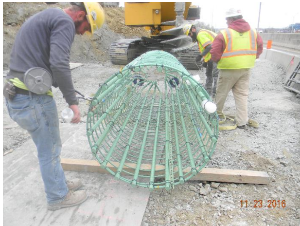
Figure 10. Installing strain gages in the drilled shafts.
