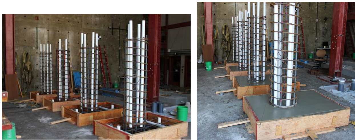
Figure 2.10 – Casting the footings
