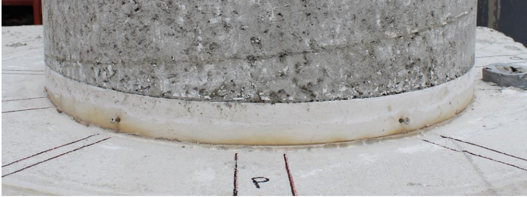
Figure 3.25 – Bottom of Pile Specimen #12
