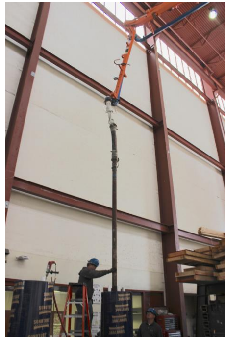
Figure 2.12 – Concrete placement using pump-fed tremie
