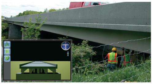
MDOT's new 3D BRIDGE app for mobile phones and tablets (inset) allows bridge inspectors to record precise observations on a 3-D model of the bridge during inspection.
