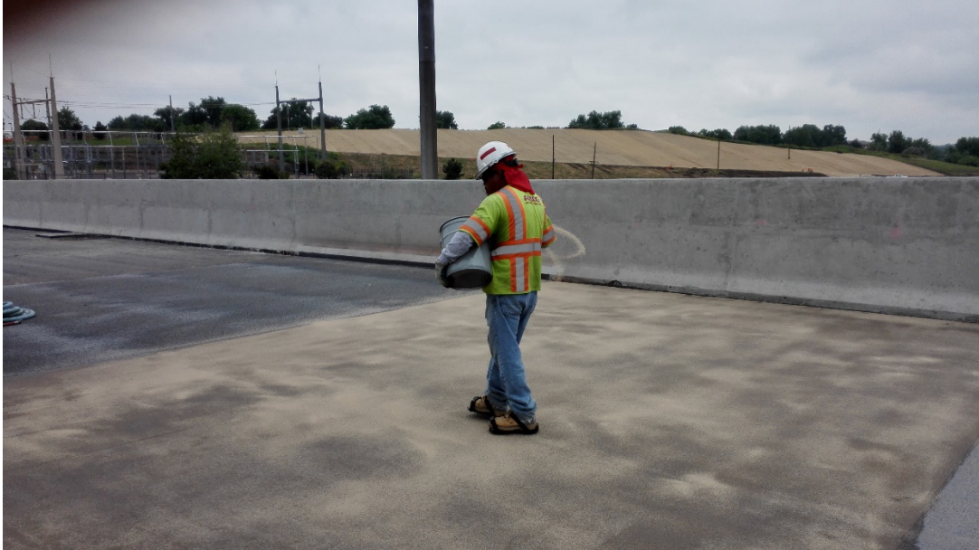
Figure 4-8. Installation of Sikadur waterproof membrane
