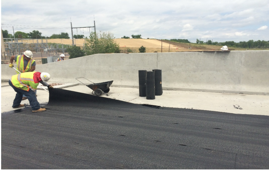
Figure 4-10. Installation of hot mix control section
