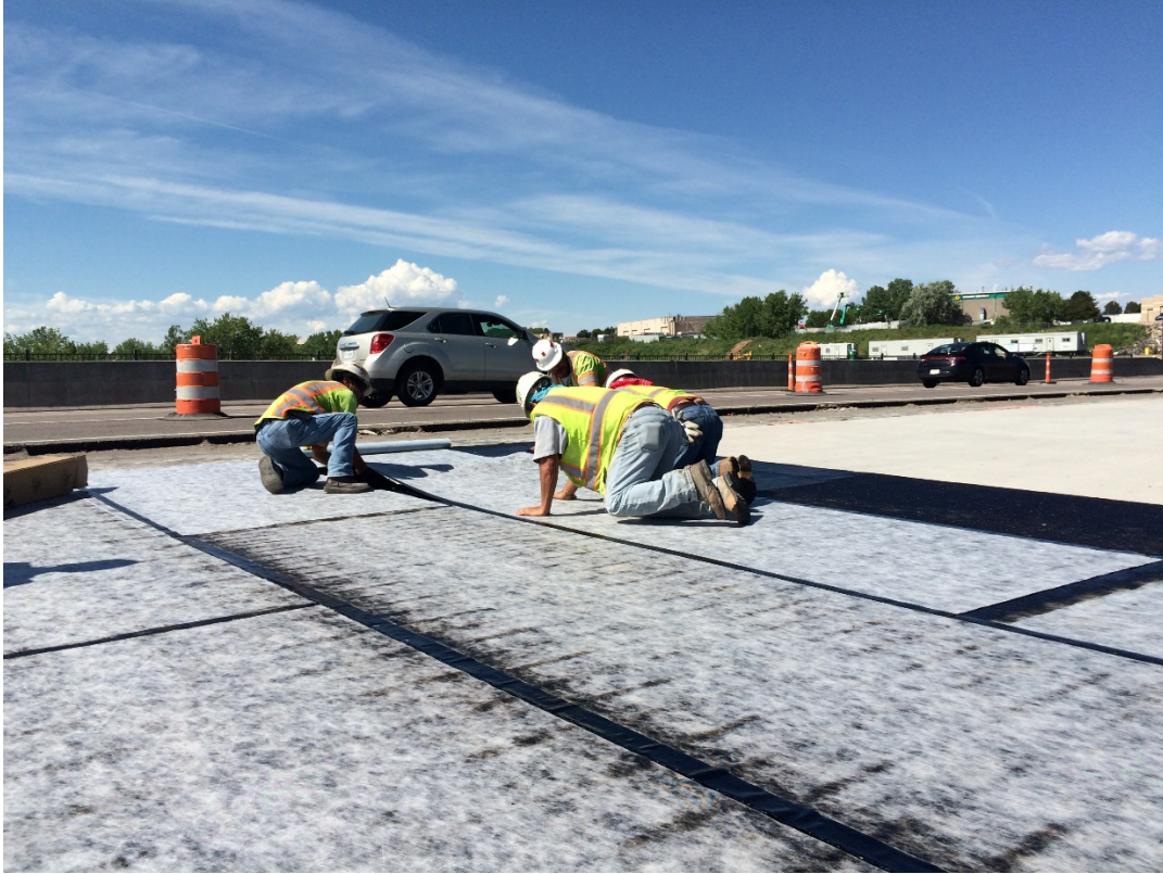
Figure 4-6. Installation of Protecto Wrap waterproof membrane
