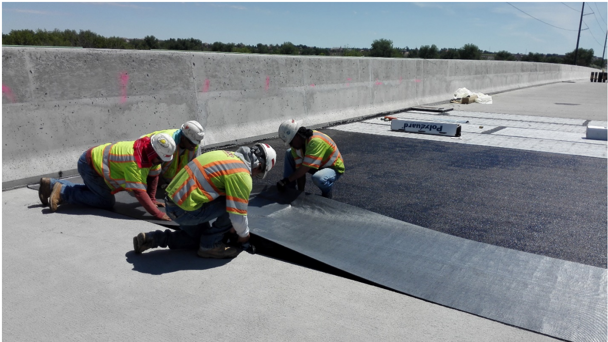
Figure 4-7. Installation of Polyguard waterproof membrane
