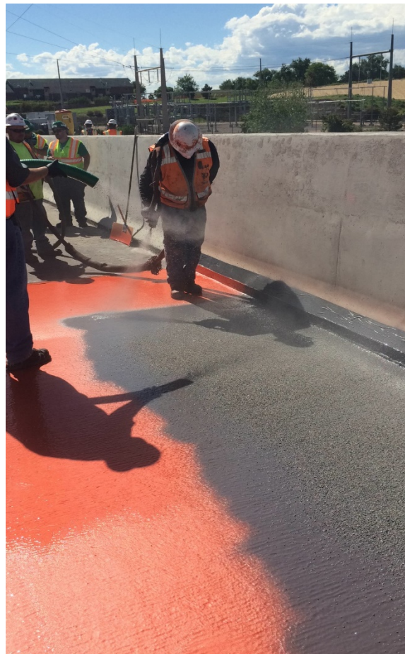
Figure 4-9. Installation of Bridge Preservation™ waterproof membrane
