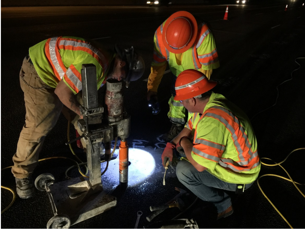
Figure 4-12. Drilling concrete cores
