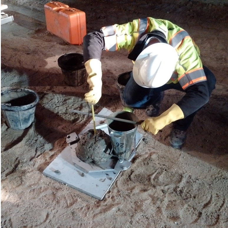
Figure 4-3. Slump test before casting the concrete
