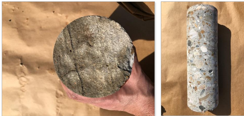
Figure 8: Core from one of the Replacement Panels
