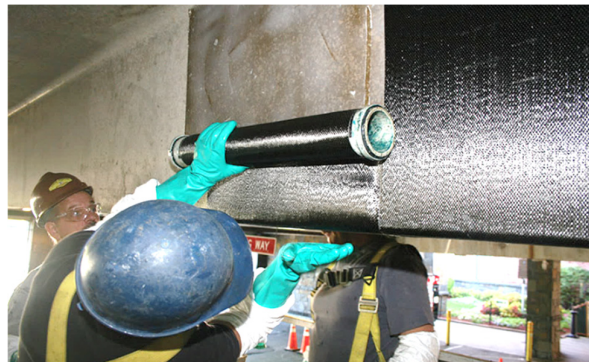
Figure 12. Bonded CFRP strips used to strengthen concrete structure [30]
