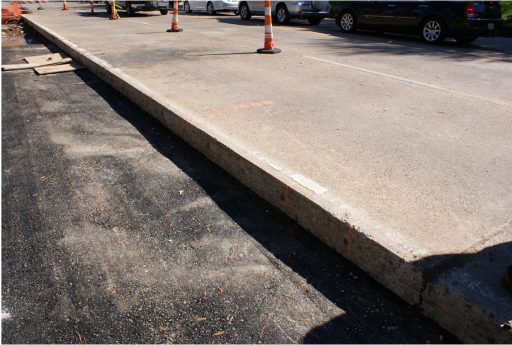
Figure 4. Photo. Short section of ATB next to existing pavement.
