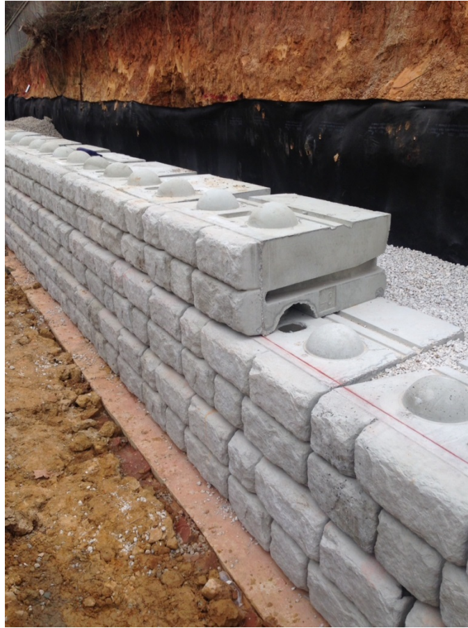
Figure 7. Photo. Wall with three courses of block installed.
