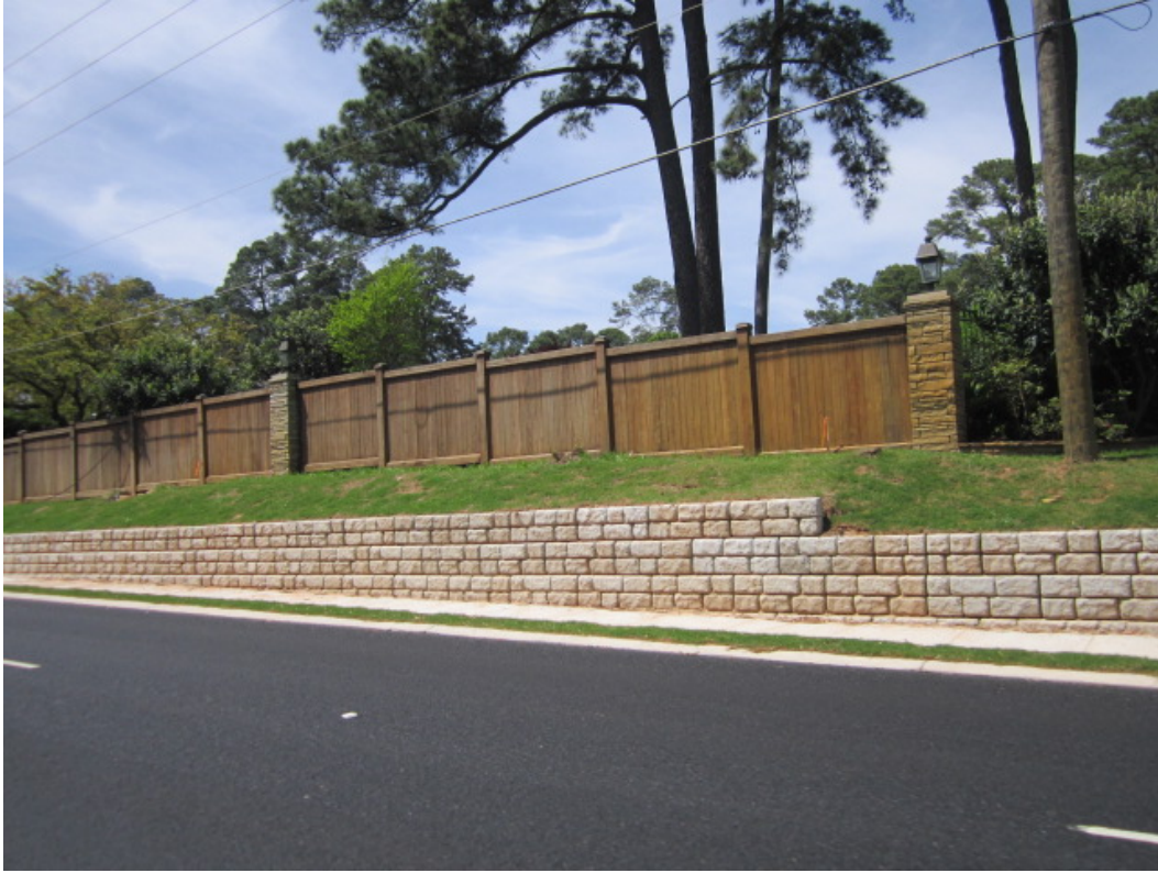
Figure 8. Photo. Completed gravity retaining wall system.
