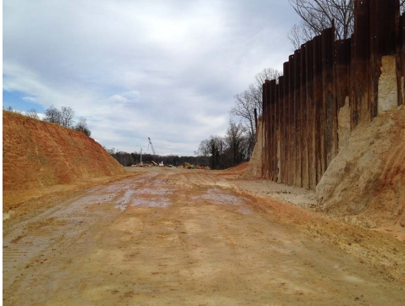
Figure 2-3 View of site after 22-ft excavation
