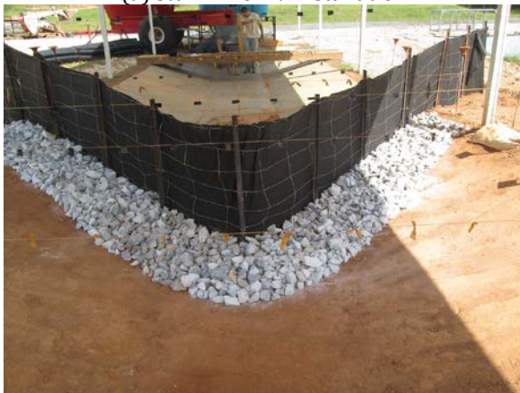
(c) std. ALDOT V install. w/mod. #4 dissipater
