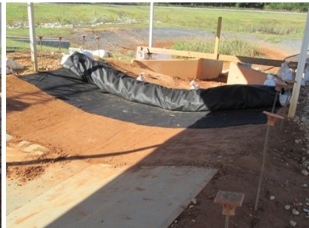
(b) Filter fabric "burrito" method
