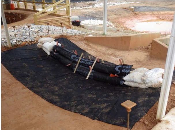
(a) Erosion Eel stacked installation
