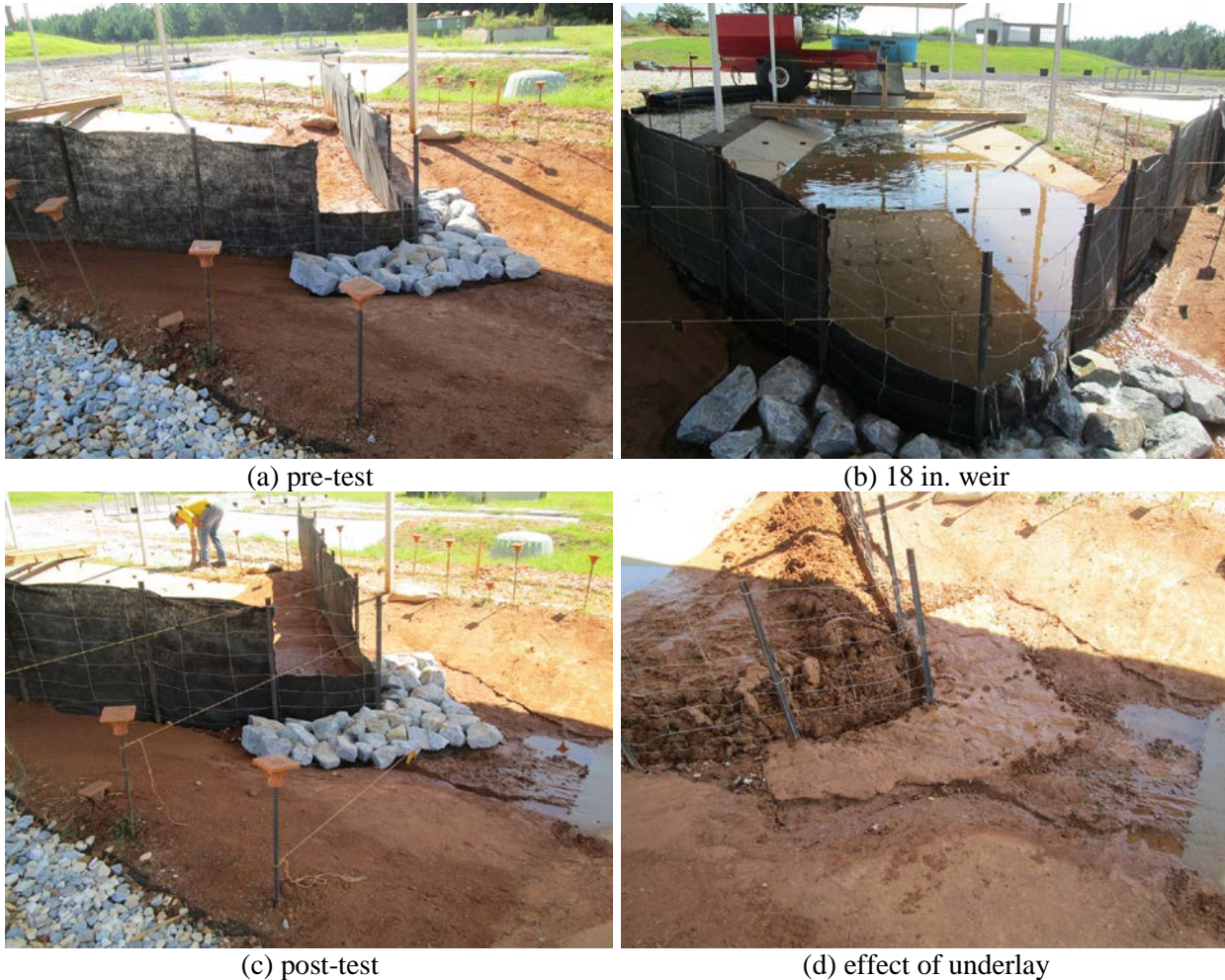
Figure 5.6: TDOT Enhanced Silt Fence Ditch Check Test.
