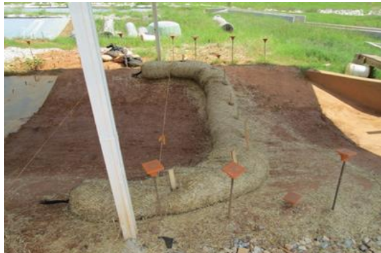
(f) Downstream Staking w/Trenching
