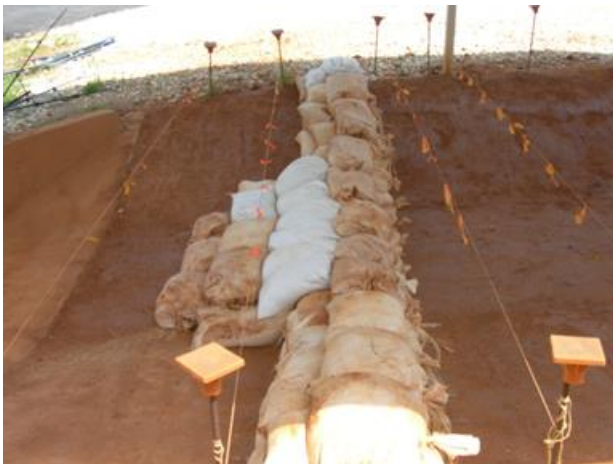
(a) downstream reinforcement sand bags
