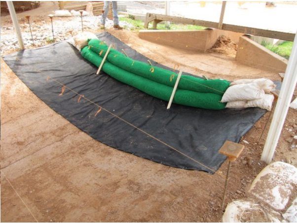
(b) Filtrexx Filter Soxx stacked installation
