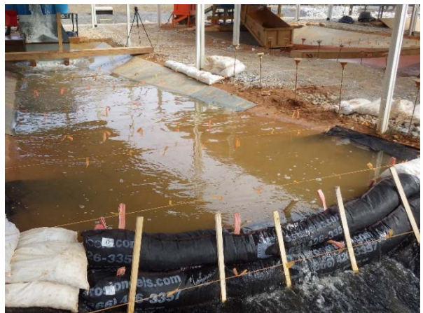
(e) Erosion Eel clean water at 1.12 cfs
