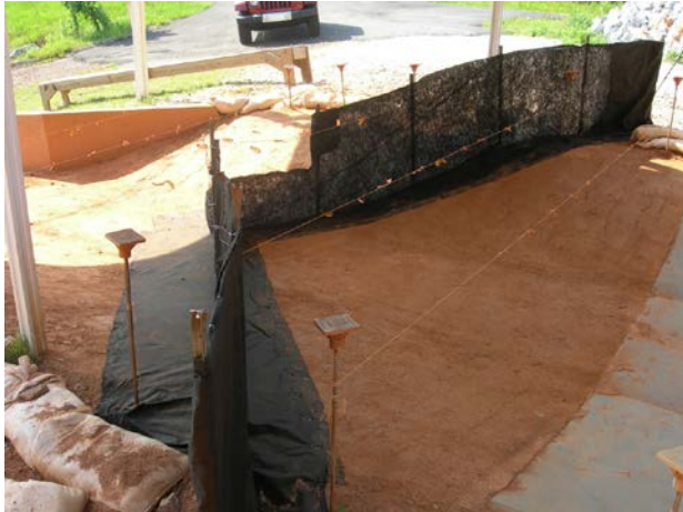
(a) FF underlay and pinning of fence
