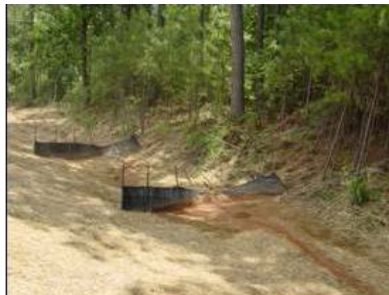
(b) ditch check under channelized flow
