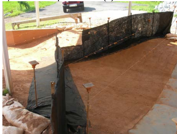
(e) enhanced ALDOT pinned installation
