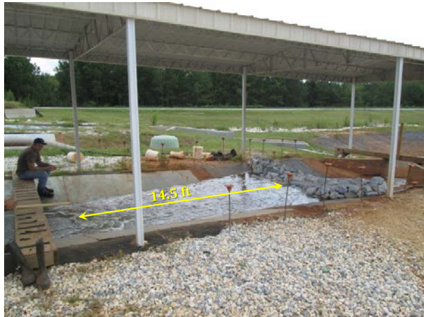
(a) Riprap ditch check w/no choker
