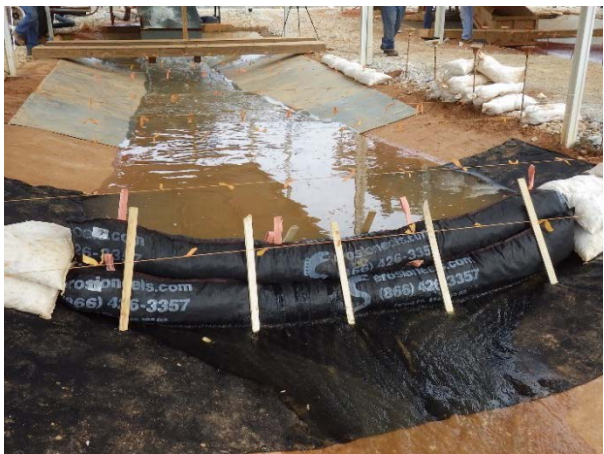
(c) Erosion Eel clean water at 0.56 cfs
