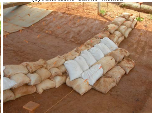
(d) Addition of downstream support bags
