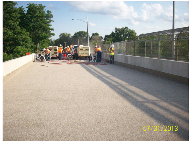
Second layer deck preparation on the Johnson County bridge deck
