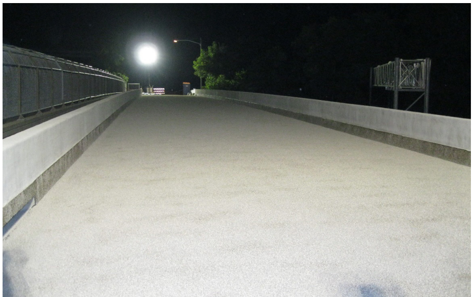
First polymer layer complete on the Johnson County bridge
