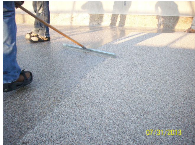
Spreading second layer of polymer on the Johnson County bridge deck
