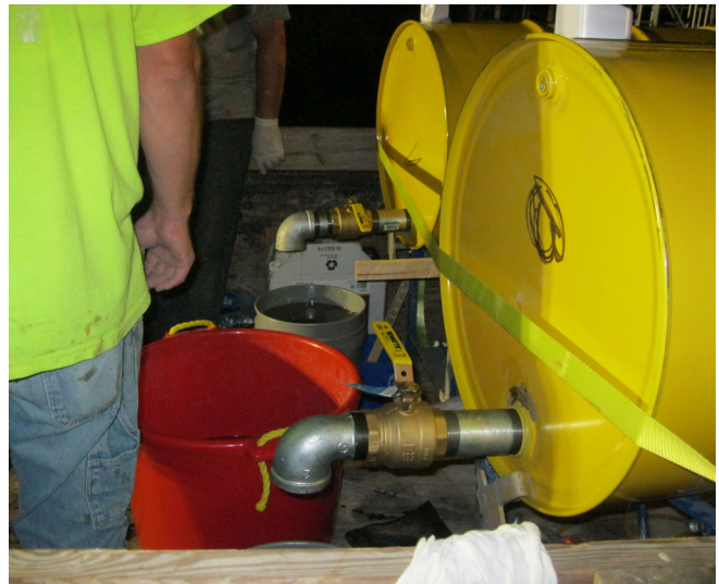
Two-part epoxy polymer mixing for the Johnson County bridge deck
