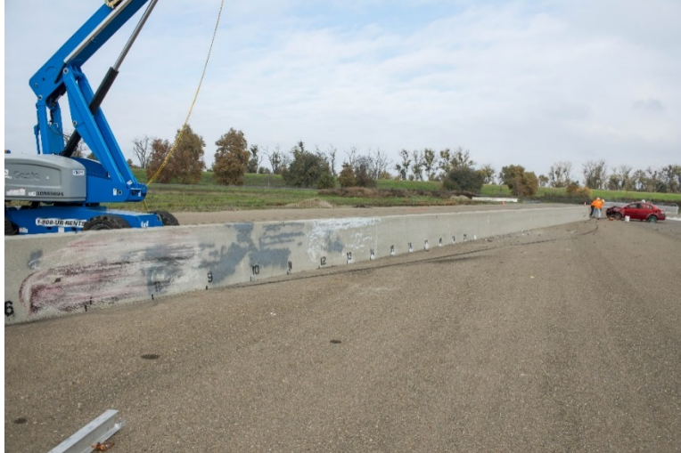
Figure 5-8 Type 60 Barrier Post-Test Downstream of Impact
