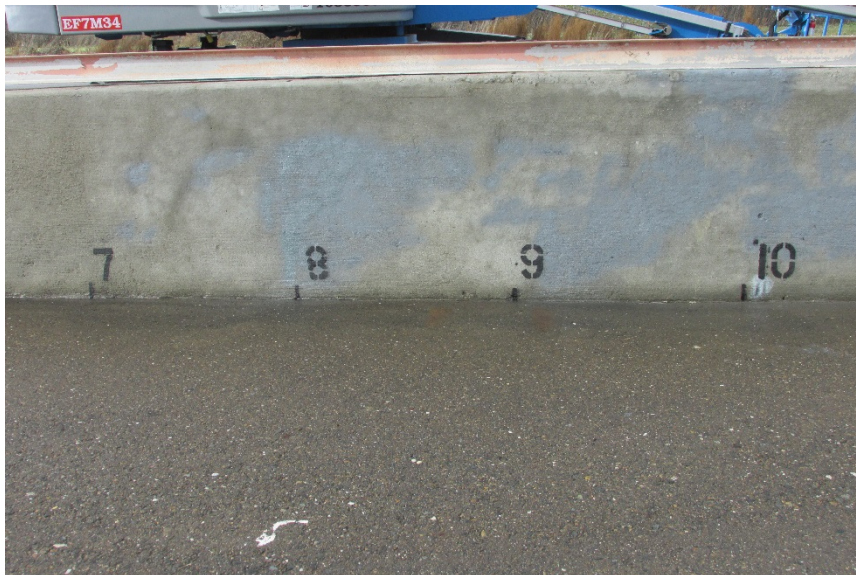
Figure 5-3 Barrier Face Downstream of Impact (I-beam on barrier was removed prior to test)
