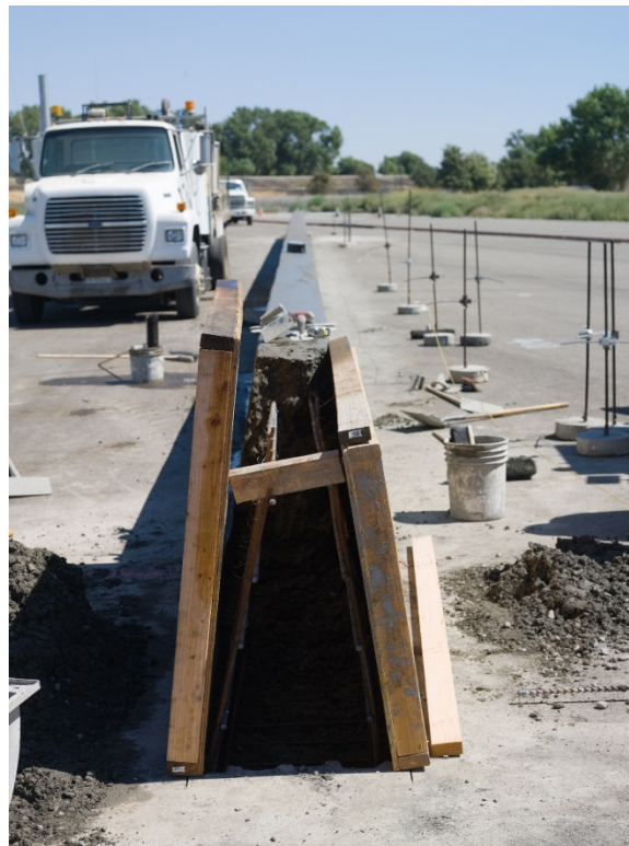
Figure 2-7 Formwork and Steel in Place for End Anchorage
