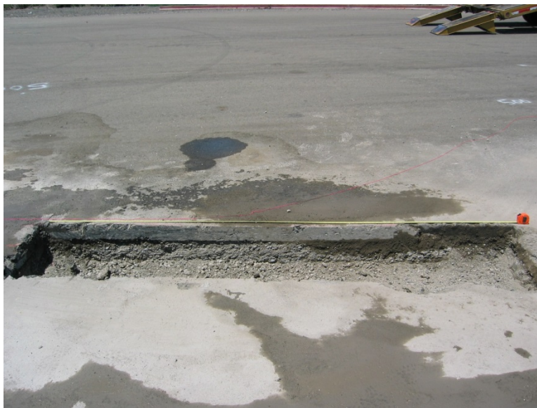
Figure 2-1 Asphalt and Aggregate Base Removed for End Anchorage Footing
