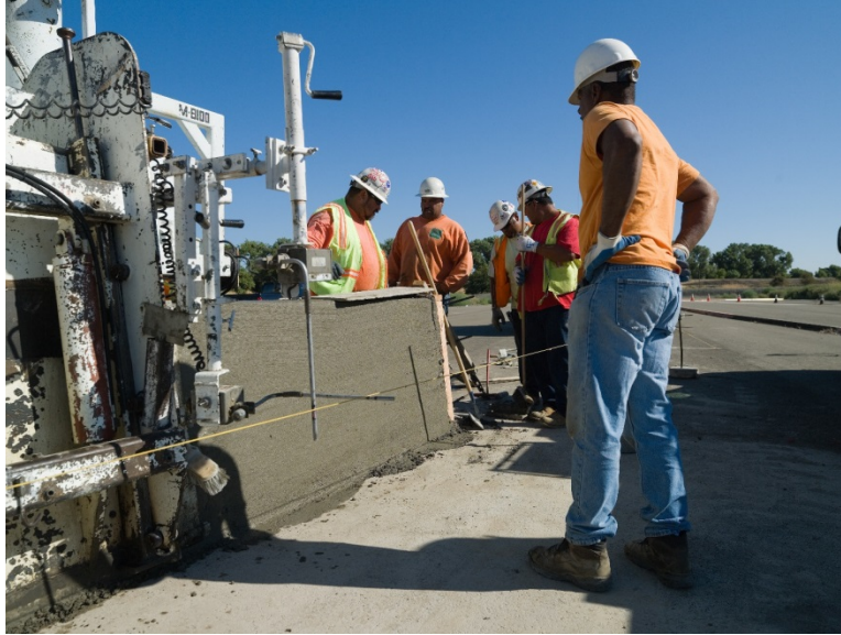
Figure 2-4 Slip-forming the Barrier
