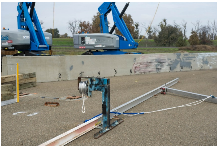
Figure 5-7 Type 60 Barrier Post Test Upstream of Impact
