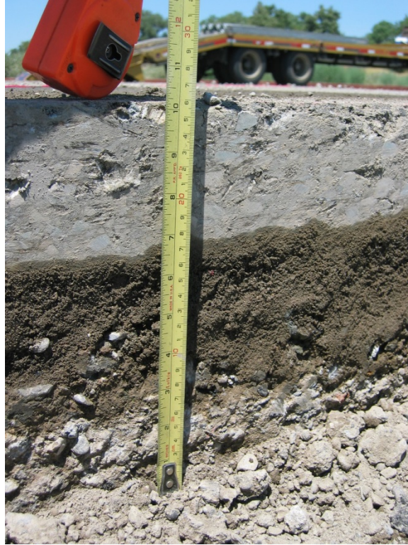
Figure 2-2 Footing Depth
