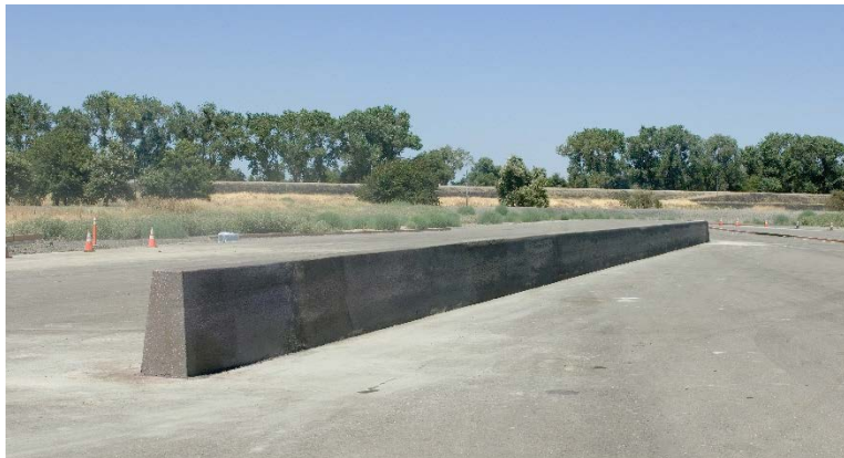
Figure 2-9 Completed Test Article: Concrete Barrier Type 60
