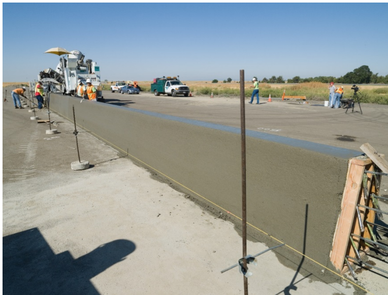
Figure 2-5 Slip-forming Nearly Complete
