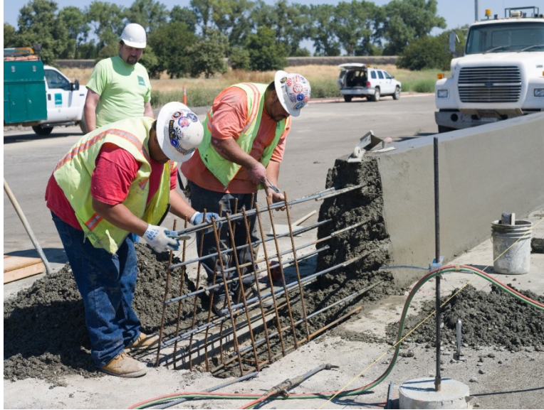
Figure 2-6 Placing Rebar for the End Anchorage
