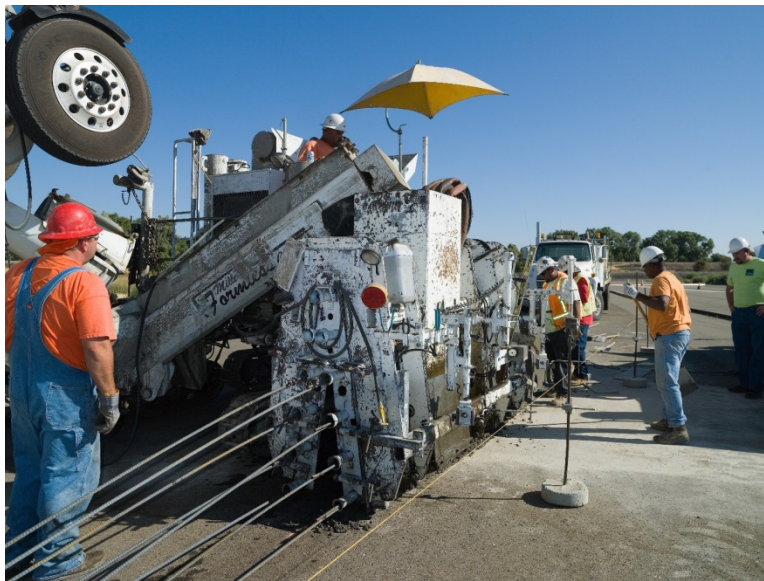
Figure 2-3 Beginning of Slip-forming
