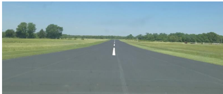
Figure A.19. Test Location at the Buffalo Municipal Airport (Google)
