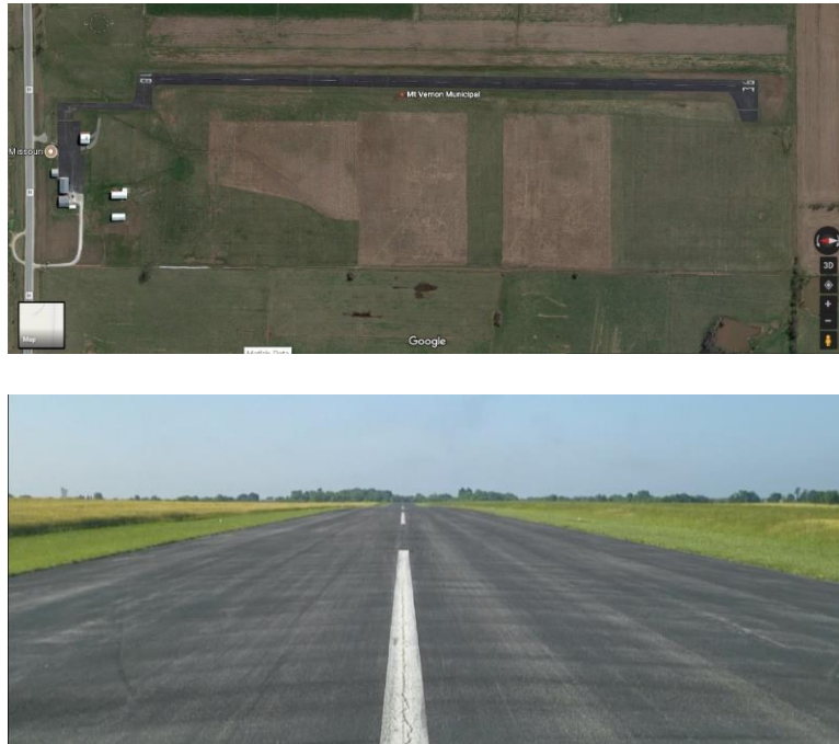
Figure A.58. Test Location at the Mount Vernon Municipal Airport (Google)
