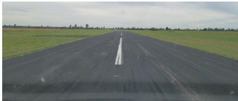
Figure A.46. Test Location at the Hornersville Memorial Airport (Google)
