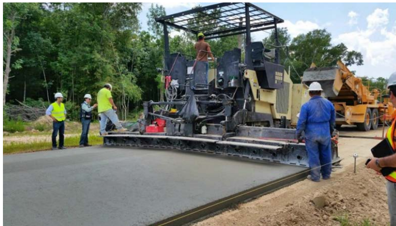
Figure 1. High-density paver placing RCC pavement from Prusinski (2016).
