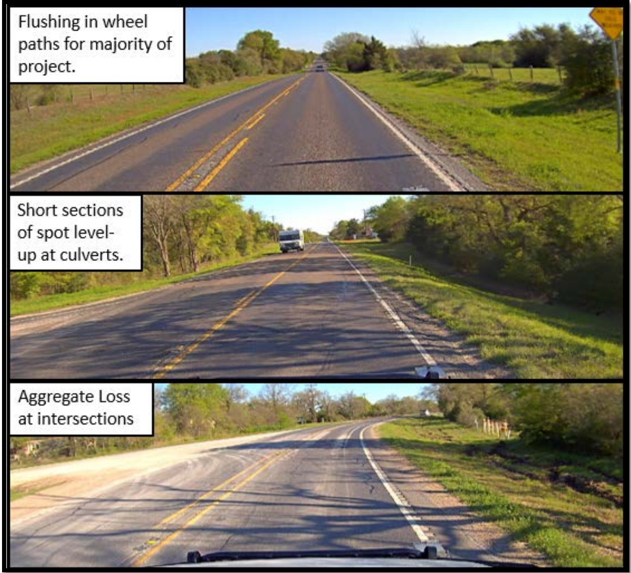
Figure 23. FM 60 Eastbound Surface Conditions.
