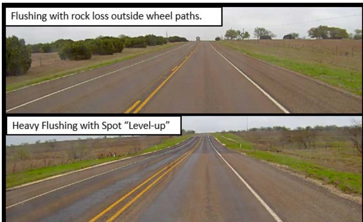
Figure 31. FM 2490 Surface Conditions.
