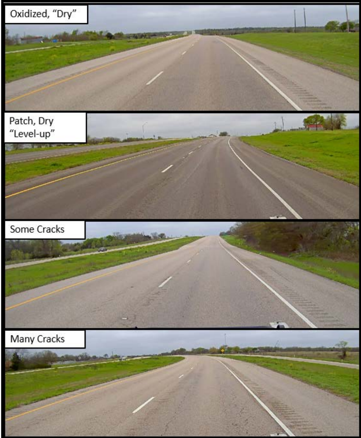
Figure 34. SH 31 Surface Conditions.
