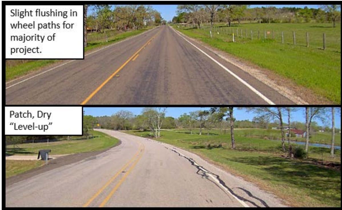
Figure 22. FM 1774 Surface Conditions.
