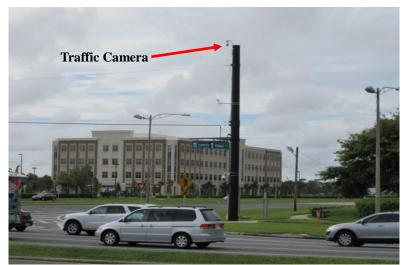
Figure 11: Traffic camera on top of mast arm support at Kirkman road and I-Drive
