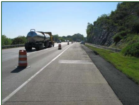
Figure 2. Eastbound view of the incident site.
