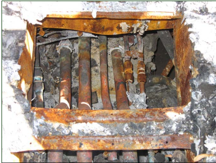
Figure A-13. View of the rear aisle area looking rearward.
