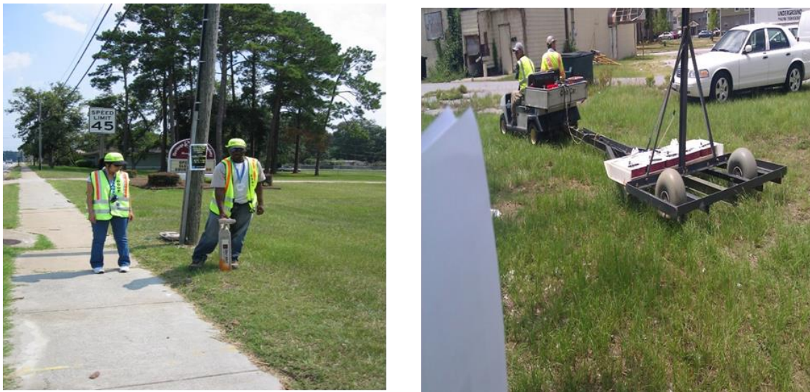
Figure 7 Geophysical Location Methods (Quality Level B) (Provided by GDOT Utilities Office)
