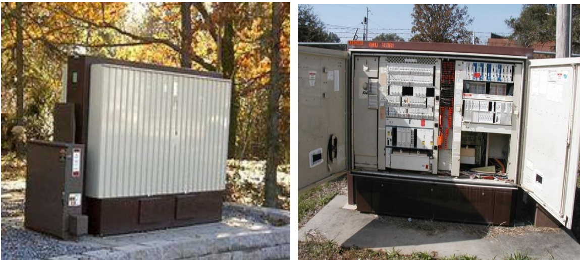
Figure 3 Subscriber Loop Carrier (Provided by GDOT Utilities Office)
