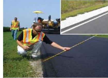
B. Safety Edge SM aids drivers in returning to pavement. (27)
