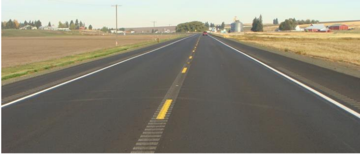
A. Shoulder and center line rumble strips alert drivers to a drift. (26)
