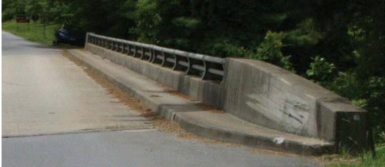
Figure 1. Unshielded bridge rail end
