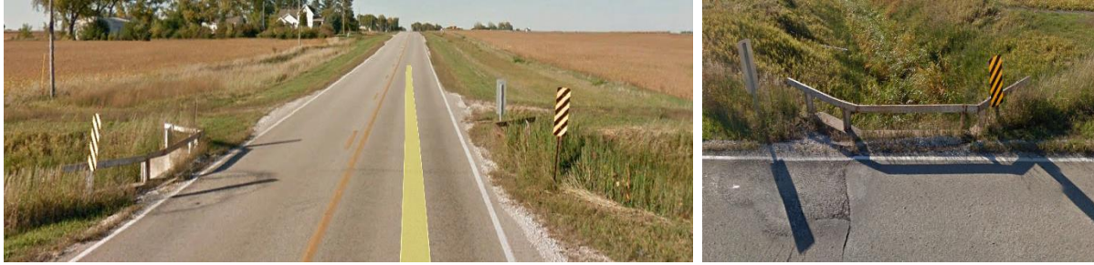
Figure 2. Example of a bridge structure struck more than once
