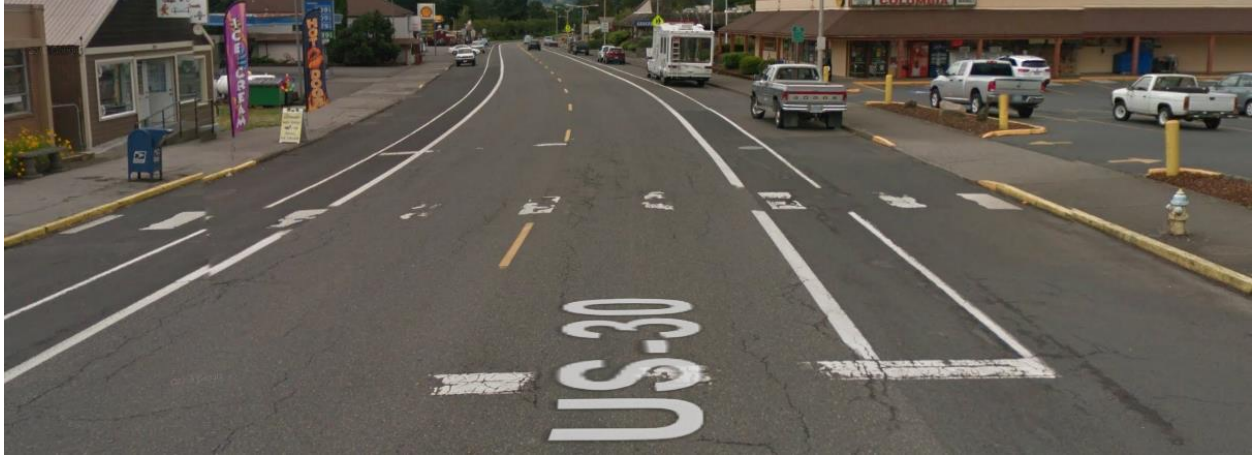
Figure 5.24: Wa Na Pa St. and SW Regulator St.
