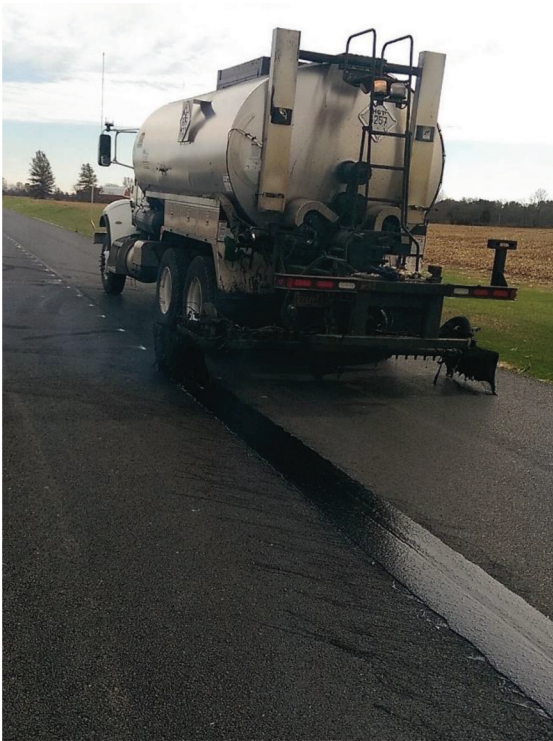
Figure 3.4 VRAM application on SR 26 in Indiana.
