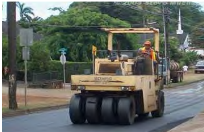
Figure 6 - Rubber Tire Roller for Embedding Aggregates [9]
