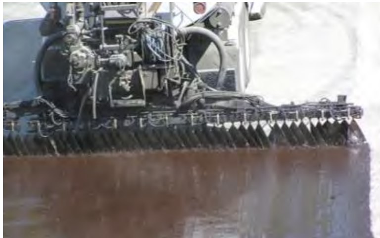
Figure 4 - Truck Mounted Sprayers for Oil distribution over the Pavement Surface [7]
