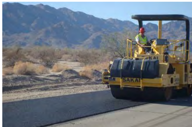
Figure 9 - Compaction of Asphalt Overlay [20]
