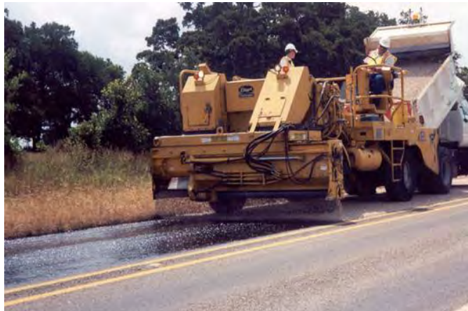
Figure 5 - Aggregate Spreader Distributes Aggregates Over the Coated Surface [8]
