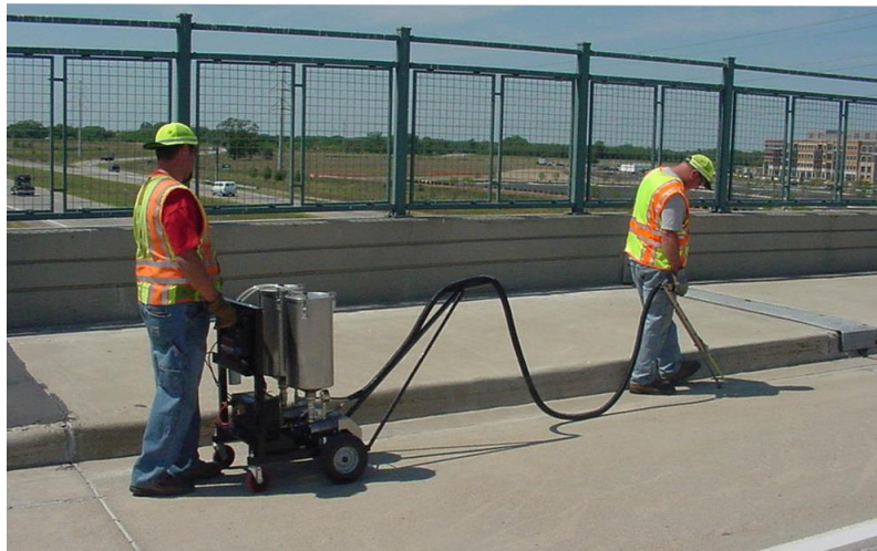
Figure 6-1 Application of Concrete Sealer (Johnson, 2009)
