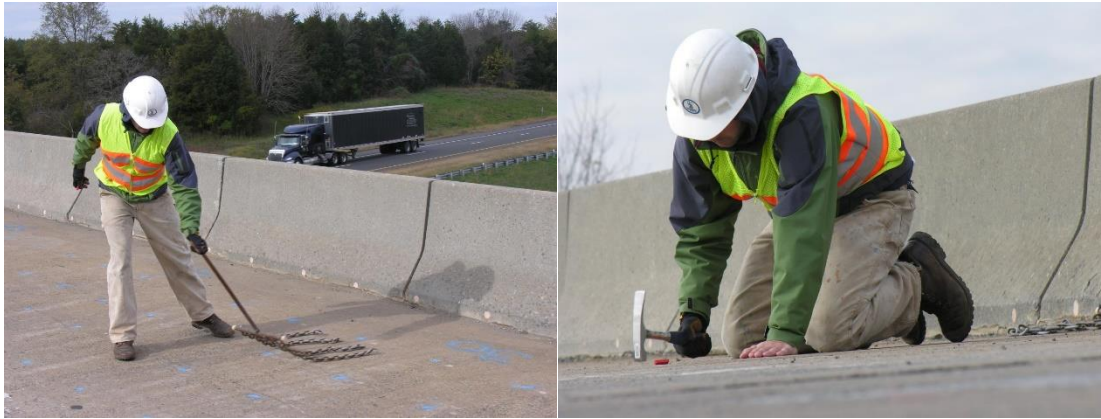
Figure 1-1 Chain Drag and Hammer Testing (SHRP2, 2012)
