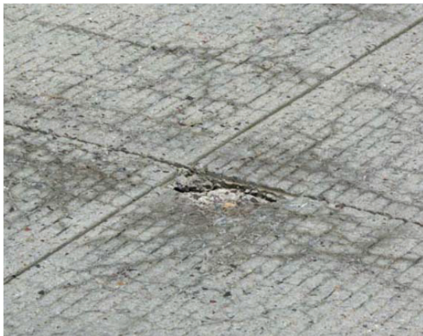
Figure A.2. Example photos showing some of the common petrographic features of ASR (cont'd). (Some of the photos are from the reference: Thomas, M.D.A., B. Fournier, and K.J. Folliard. Alkali-aggregate Reactivity (AAR) Facts Book . No. FHWA-HIF-13-019. 2013.)
