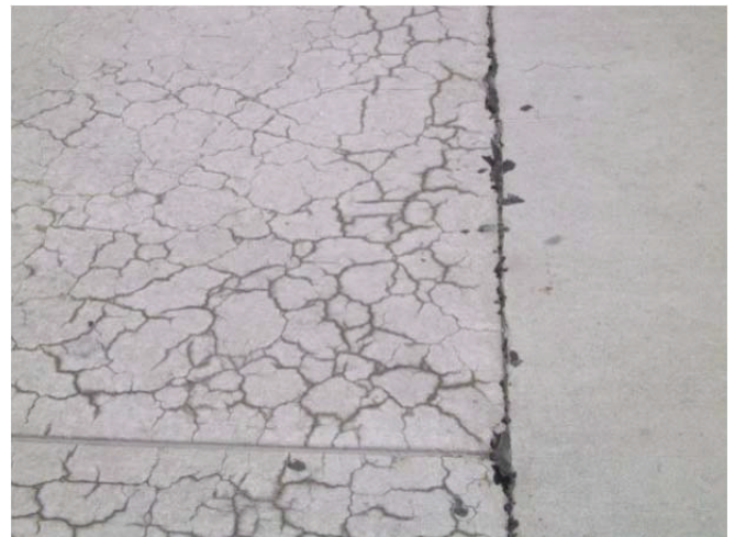
Figure A.2. Example photos showing some of the common petrographic features of ASR (cont'd). (Some of the photos are from the reference: Thomas, M.D.A., B. Fournier, and K.J. Folliard. Alkali-aggregate Reactivity (AAR) Facts Book . No. FHWA-HIF-13-019. 2013.)
