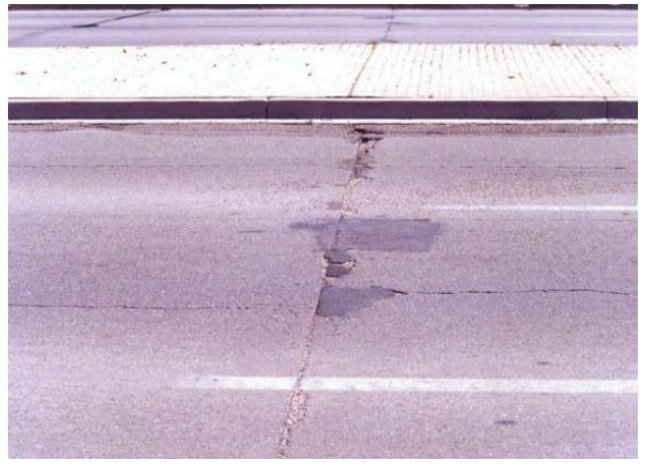
Figure A.2: Example photos showing some of the common petrographic features of ASR ( cont'd ).
