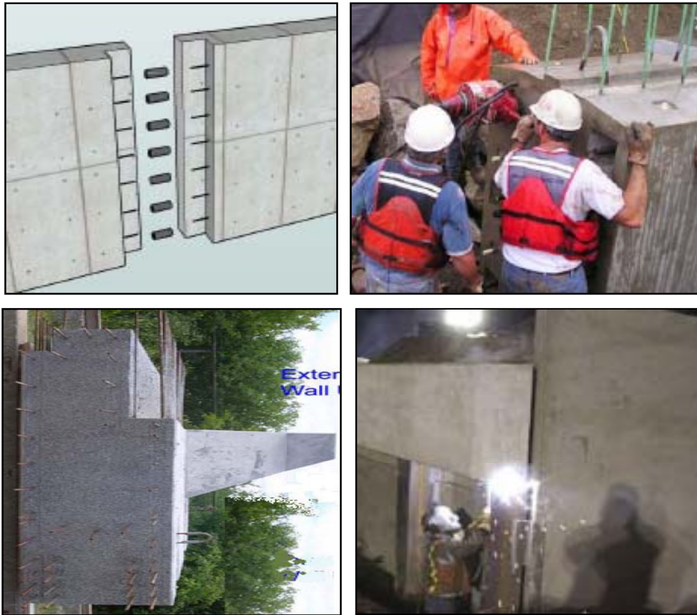
Figure 4 – Abutment module to module connection methods: Spliced Sleeves (top left), Post tensioning (6) (top right), Cast in place closure joints (7) (bottom left), Welding (8) (bottom right)
