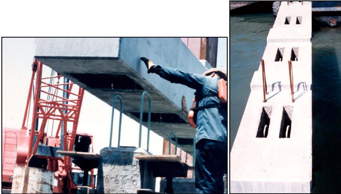
Figure 9 – Grouted Pocket Connection (14)
