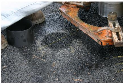
Figure 3. Installation of a 6-In-Diameter Ring in the Annular Space Following Partial Depth Coring
