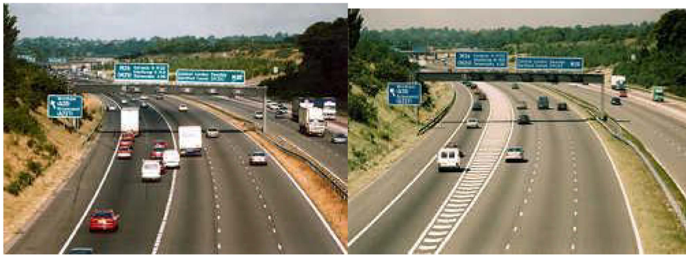
These photos show a road in England before and after it was painted with a wide striped buffer, called tiger-tail markings, to separate the merge/diverge points of each lane. (Used with the permission of the Highway Agency, UK)
