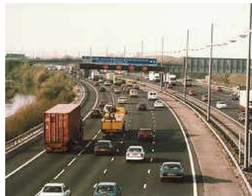
Several countries in Europe have been able to achieve considerable benefits in traffic flow and safety by changing the freeway speed limit based on real-time traffic speed and flow data. (Used with the permission of the Highway Agency, UK)
