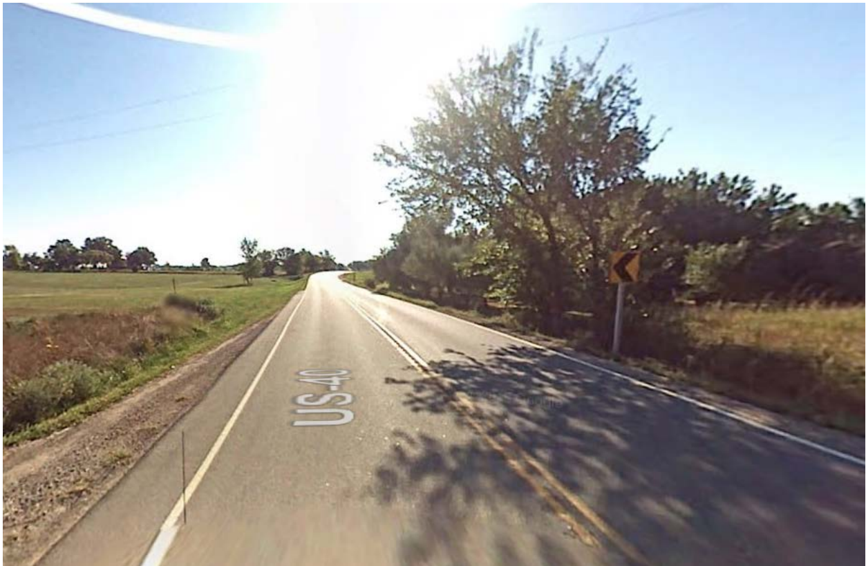
Figure 5.7: Section 20 of US-40 Showing Roadside Hazards that must be Removed to Increase Safety
