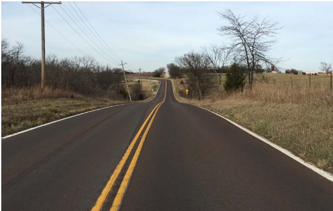
Figure 3.1: US-40 Northbound from Lawrence, KS, to Topeka, KS
