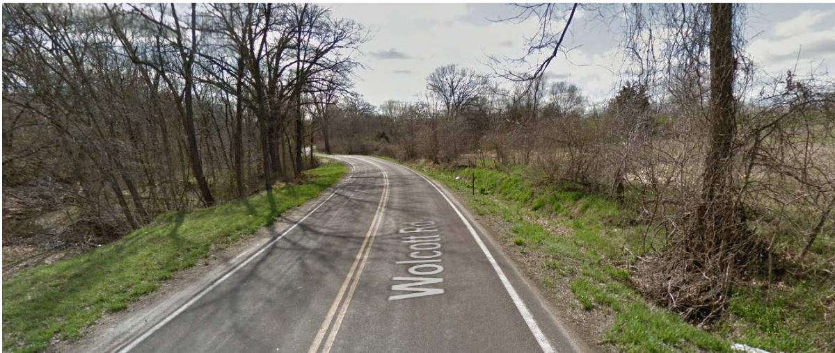
Figure 5.18: Google Street View of Two Horizontal Curves along K-5 that Require Countermeasures
