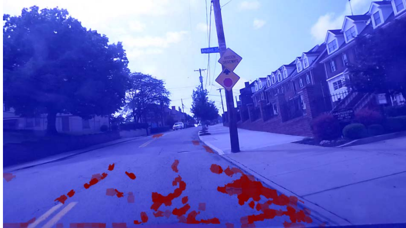
Figure 10 Classification result. The color indicates the severity of distress: blue = no cracks, red = cracks.
