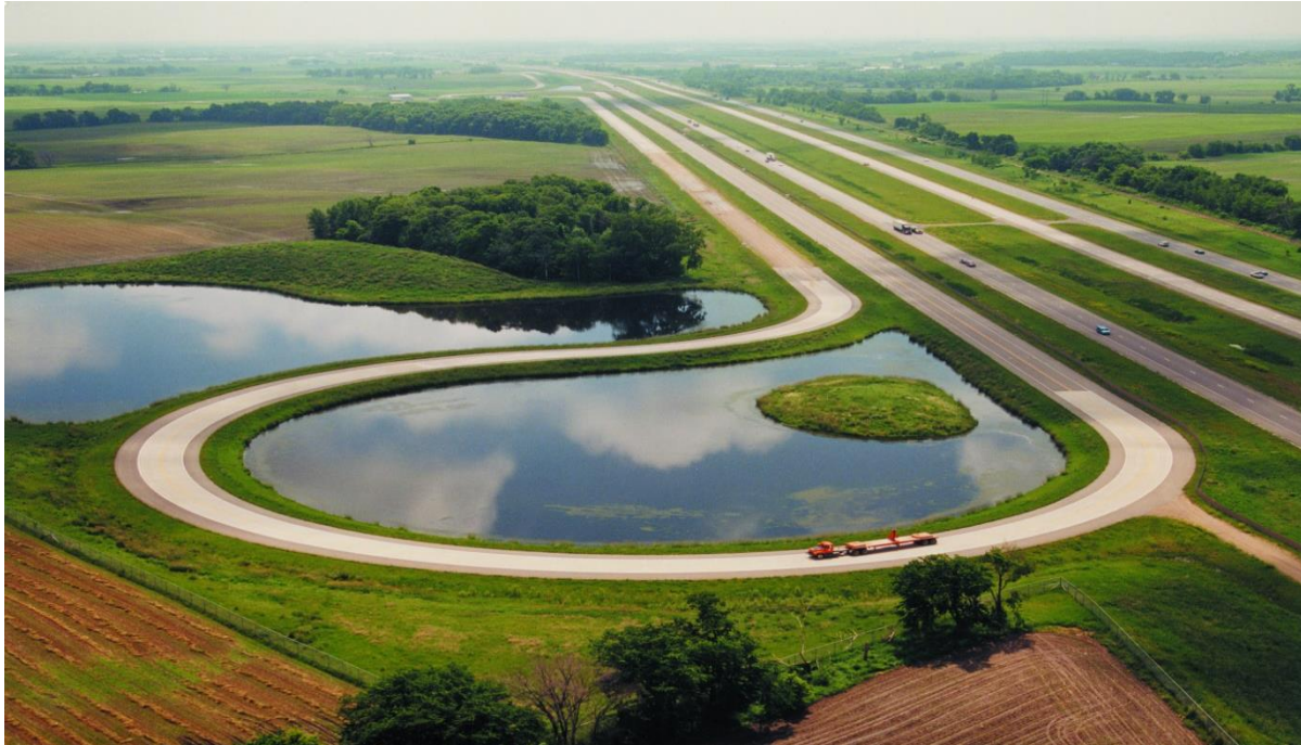
Figure 20 MnROAD road facility in Minnesota
