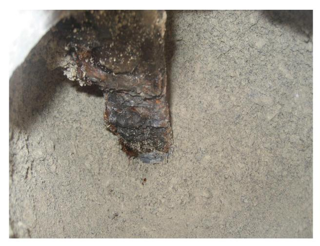
Figure 5-14: In-service galvanized soil reinforcement for I-15/ Cheyenne Blvd. Wall 1, 15 years old.
