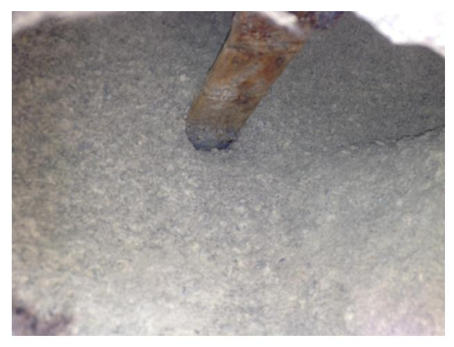
Figure 5-17: In-service galvanized soil reinforcement for I-15/ Cheyenne Blvd. Wall 2, 15 years old.
