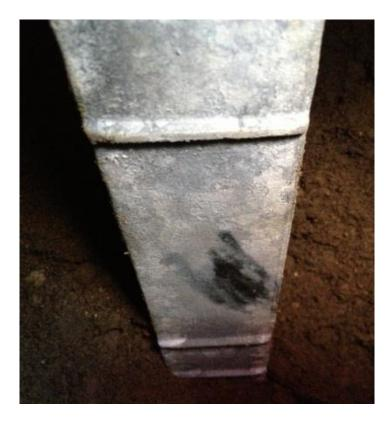
Figure 2-2: In-service galvanized reinforcement, a layer zinc carbonate can be seen along the surface. (ALT US 95 and ALT US 50, W1-SB-E1)
