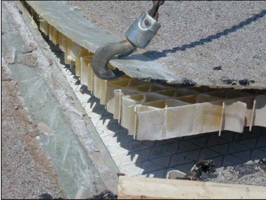
Figure 1.2: Material Delamination in Bridge Panel
