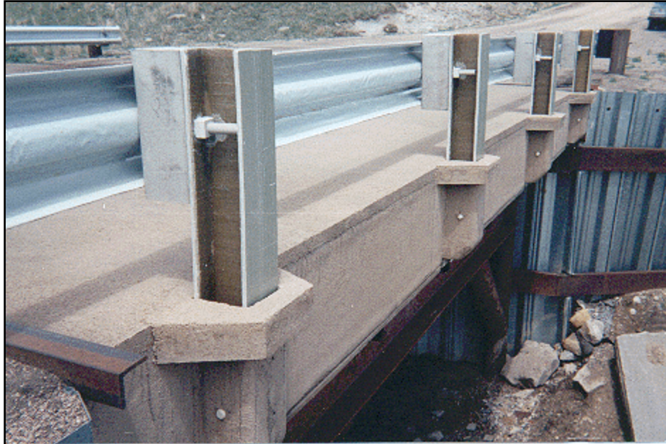
Figure 1.1: No-Name Creek FRP Bridge Source: Kansas Structural Composites, Inc. (2007)
