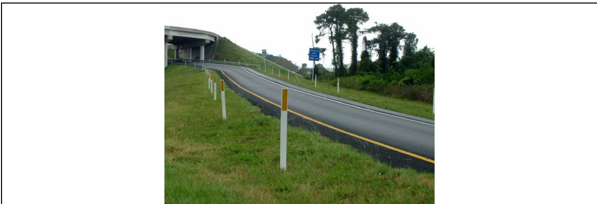
Figure 4: Post delineators used on a curve (image source: McGee and Hanscom, 2006)
