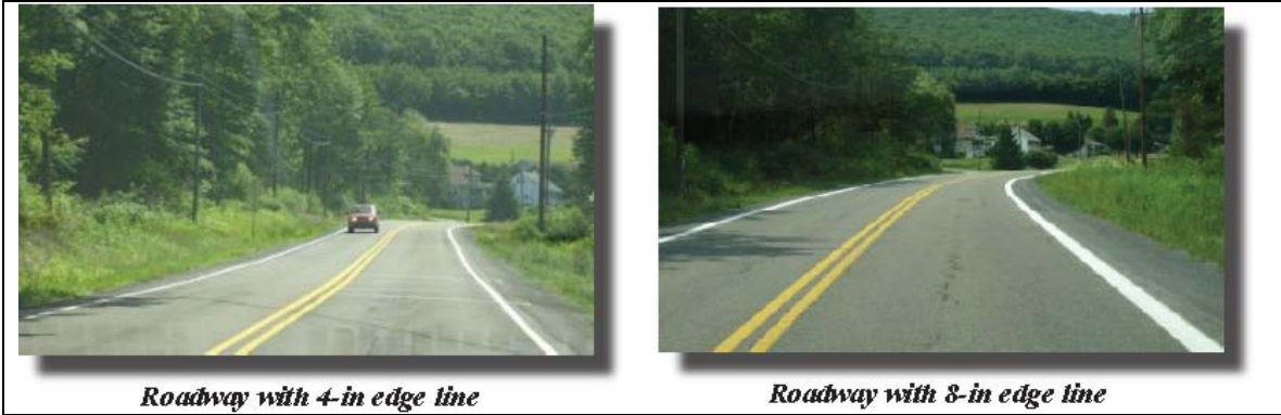
Figure 2: Use of wider edgeline on horizontal curve (image source: McGee and Hanscom, 2006)
