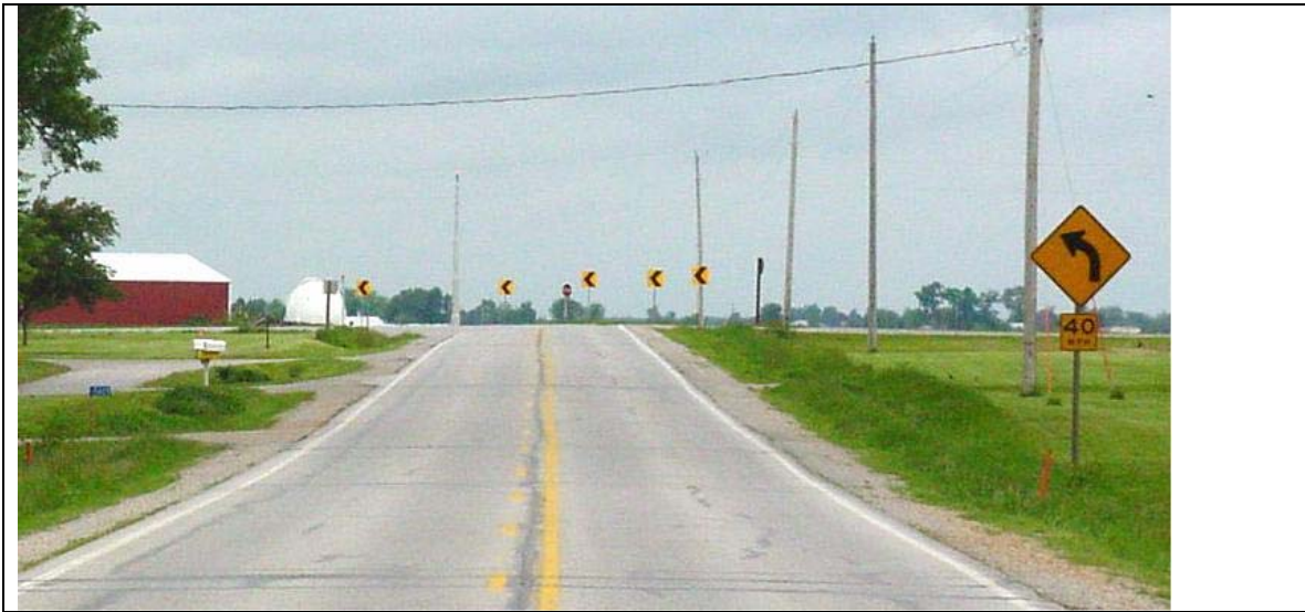
Figure 3: Larger chevrons and curve signs—US 6, Johnson County (image source: Tom Welch, Iowa DOT)
