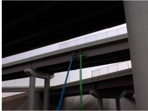
FIGURE 9 Conduit and cable installation
