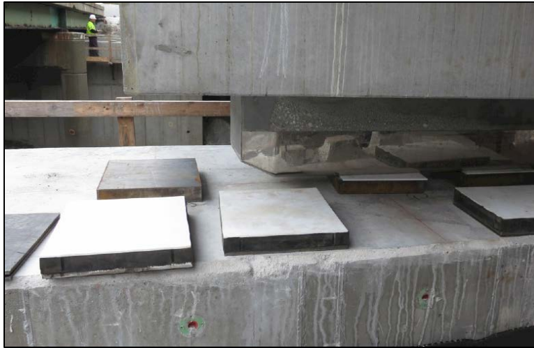
Figure 8.2. Bridge slide using PTFE sliding bearings (Source: SHRP2 Renewal Project Ro4)
