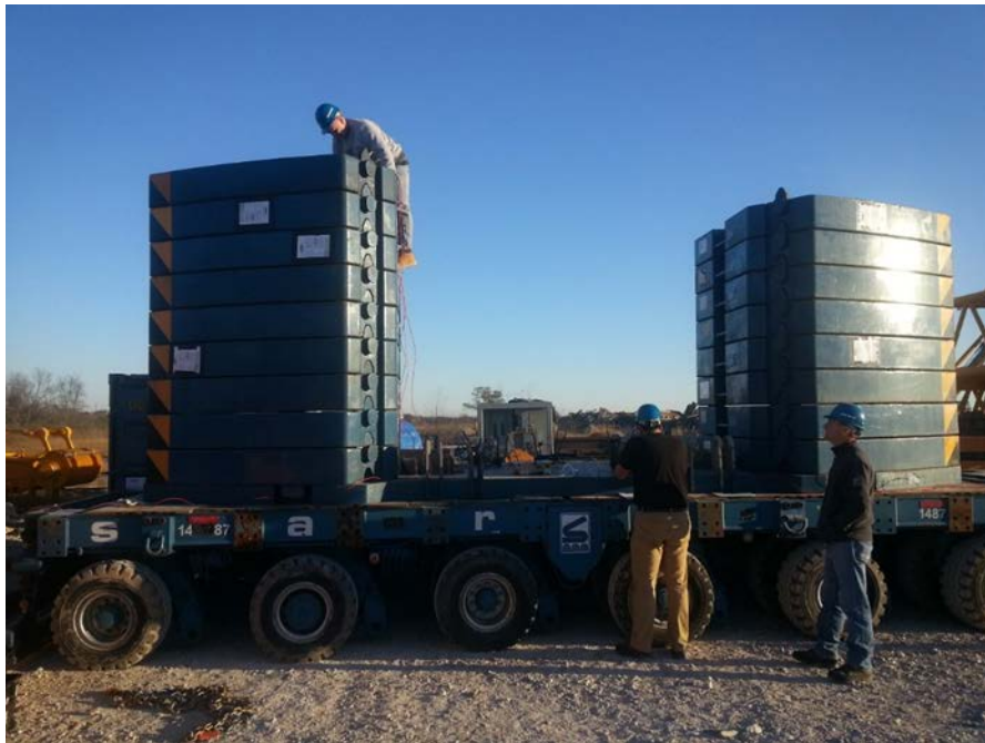
Figure 3.1. The steel weights on SPMT for heavy loading
