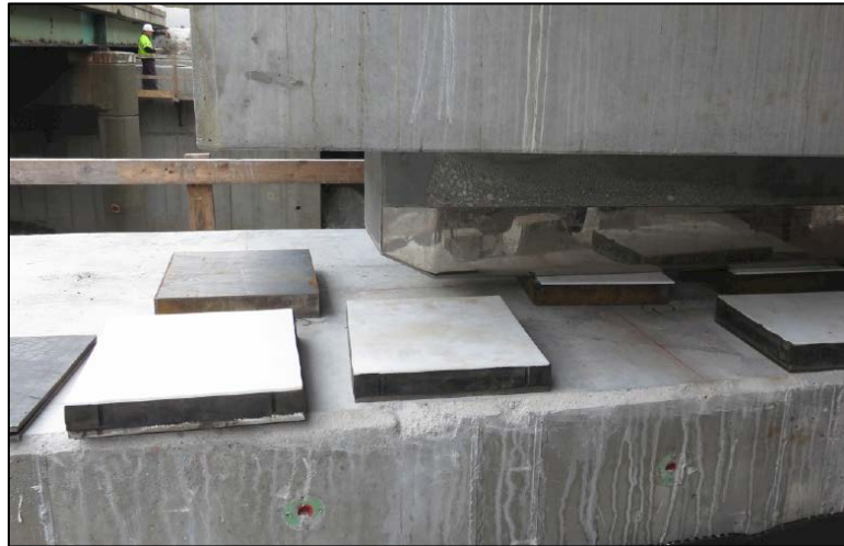
Figure 8.3. Incremental bridge launch over Iowa River (courtesy of Iowa DOT)
