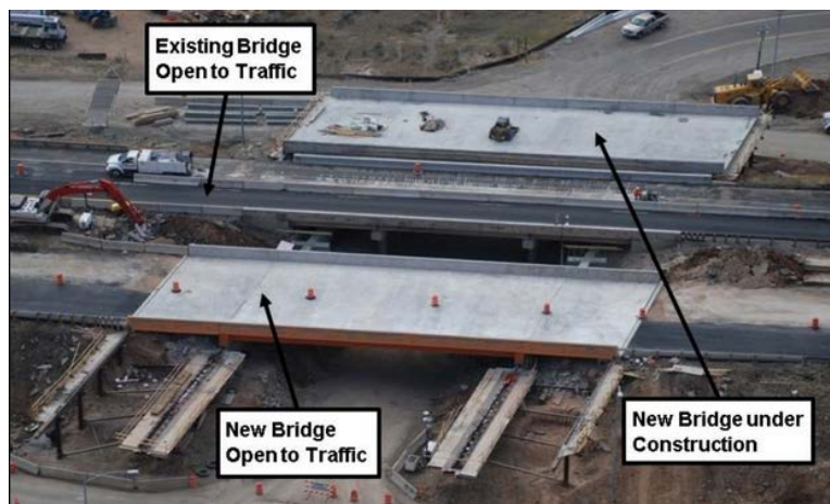
Figure 8.1. Bridge slide project in Utah (Source: FHWA Project #F-ST99(232))
