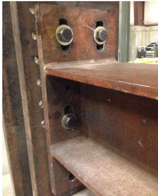
Figure 10.5. Slotted connection for spreader beam
