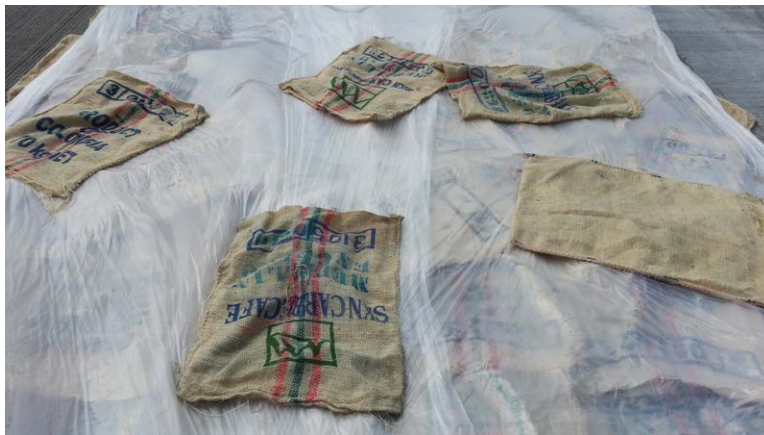
Figure 7.9 Wet curing for five days under white plastic sheets
