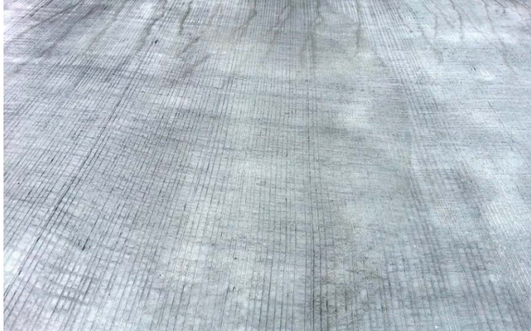
Figure 7.8 PAMS curing compound applied by the research team
