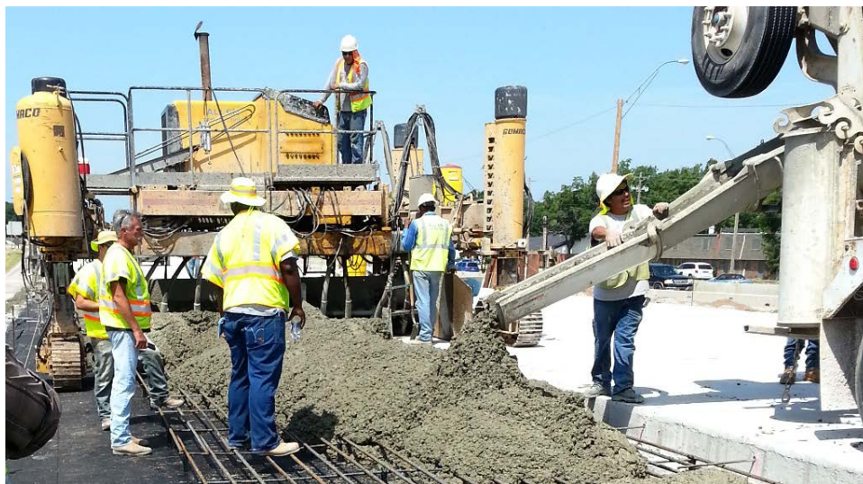
Figure 7.1 Casting the concrete pavement
