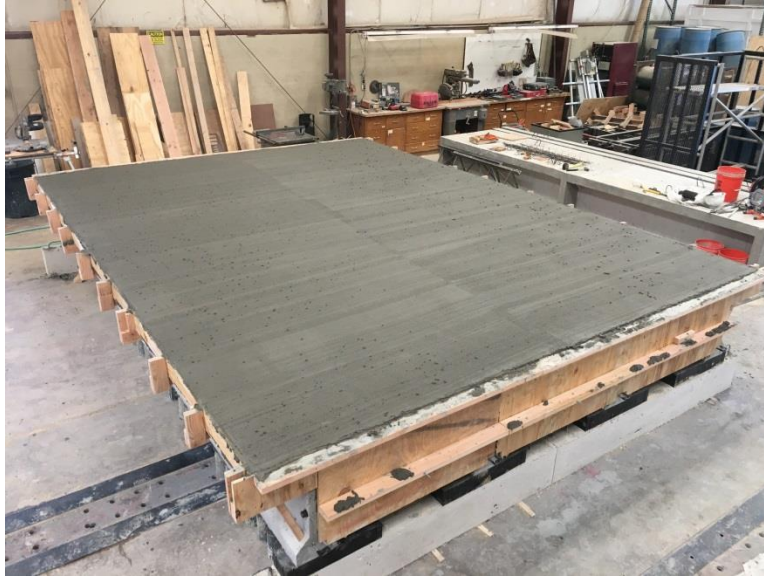
Figure 7.13: Scaled bridge deck section after concrete finishing
