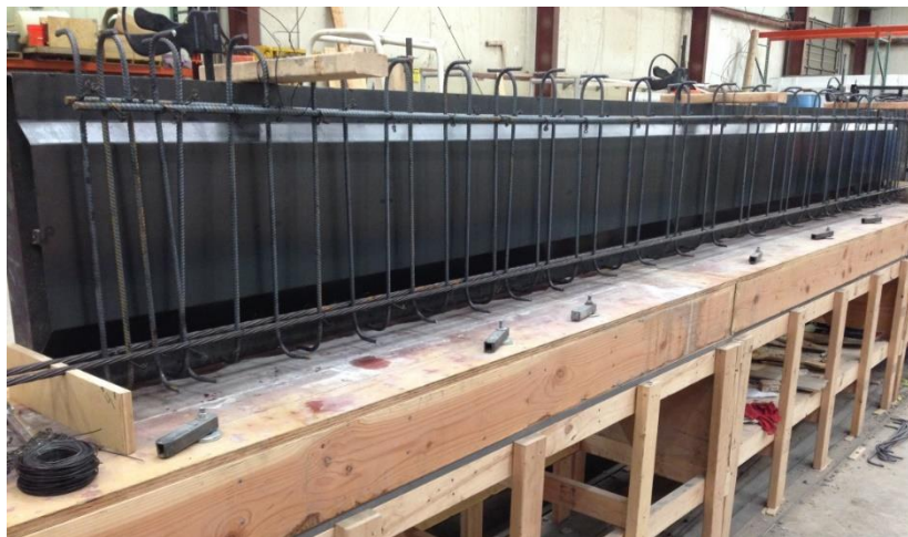
Figure 7.3. Reinforcing steel and formwork in place before beam casting
