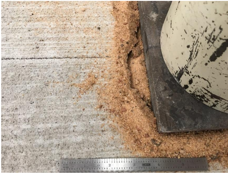
Figure 7.38: Punching shear in scaled bridge section deck at failure
