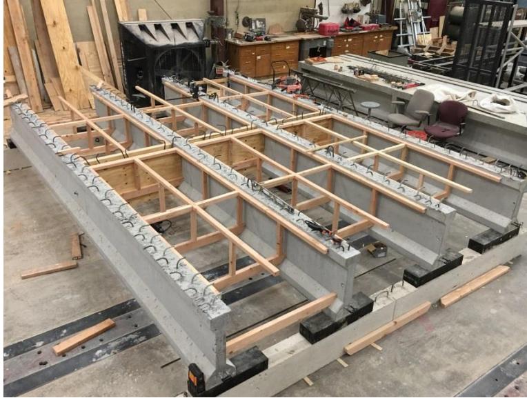
Figure 7.9: Initial framing for scaled bridge deck formwork
