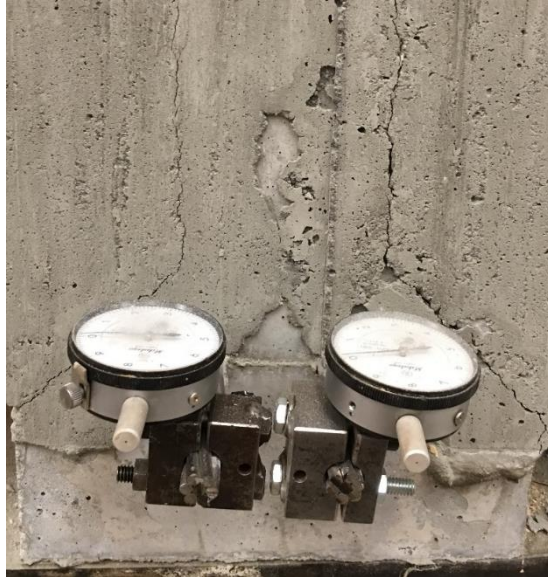
Figure 7.26: Cracking at diaphragm-girder interface
