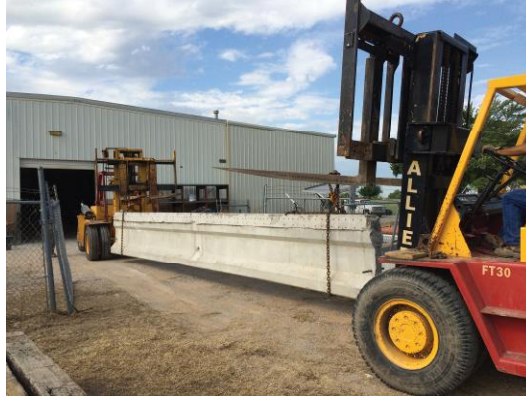
Figure 2.11: Transportation of girder A into Fears Lab on July 29, 2014
