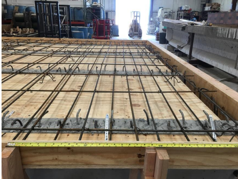
Figure 7.11: Close-up of scaled bridge deck rebar placement
