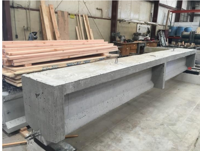
Figure 7.6: Completed scale girder C section showing end and midspan diaphragm sections
