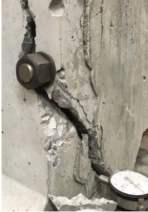
Figure 7.37: Diaphragm to girder connection at girder A4 at failure
