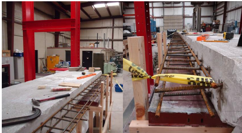
Figure 2.15: Construction of deck extension of girder C in progress
