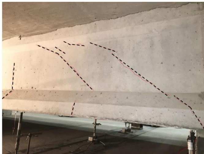
Figure 7.31: Cracking at 67 kips of load for the loaded girder
