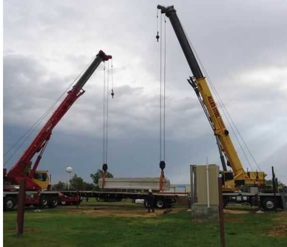
Figure 2.7: Unloading of girder A using 20 ton rental cranes on October 8, 2013
