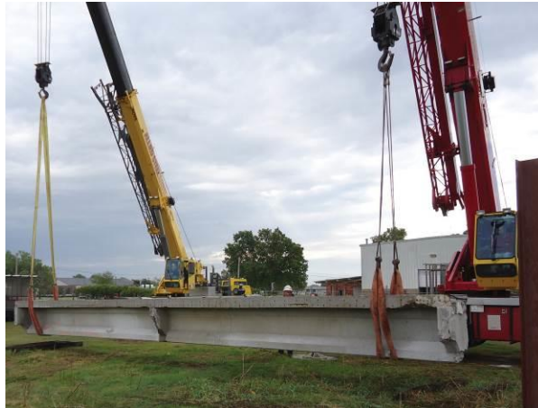
Figure 2.8: Unloading of girder C using 20 ton rental cranes on October 8, 2013
