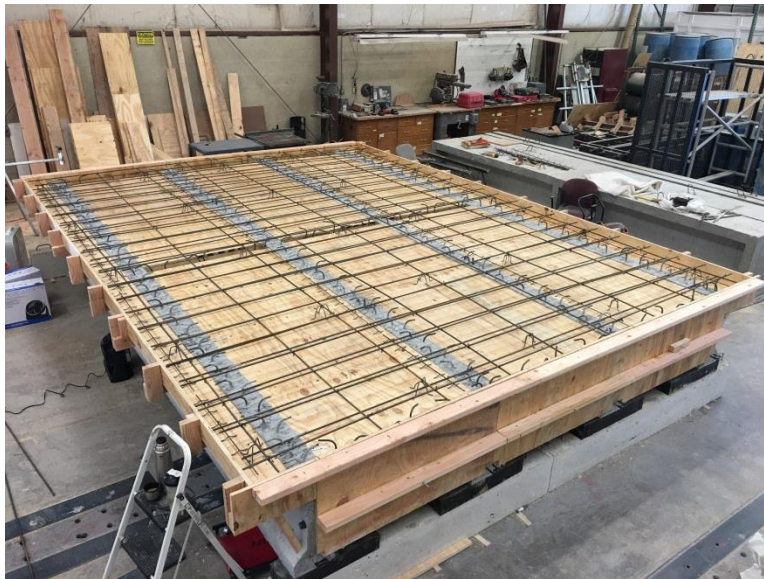
Figure 7.10: Completed scaled bridge deck formwork and rebar placement
