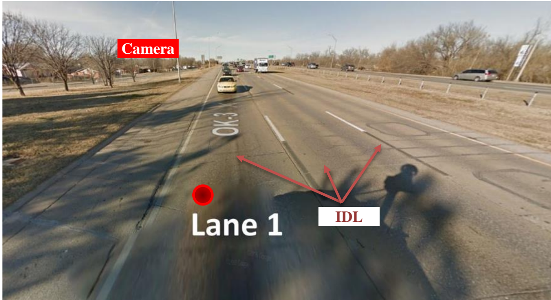
Figure 5-13 Field test 7 deployment site
