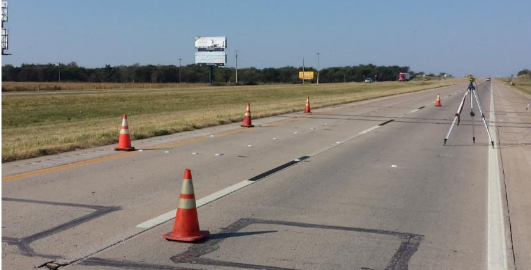
Figure 5-8 Field test 3 deployment site
