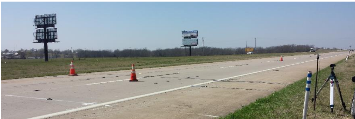
Figure 5-3 Field Test 1 deployment site
