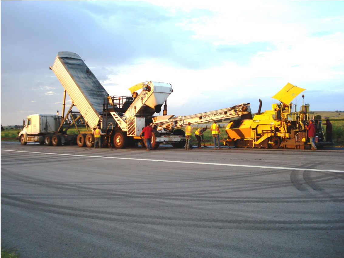
Figure 6.3. Paving Train Placing Shoulder Mix
