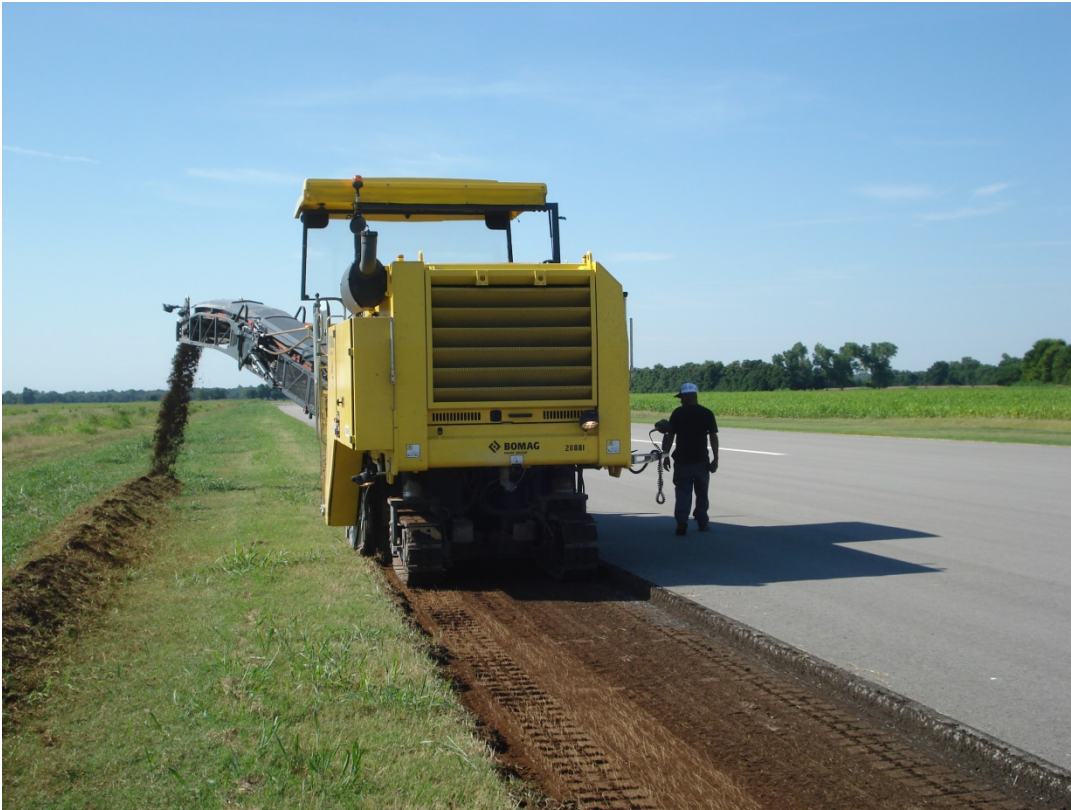
Figure 6.1. Cold Planer Excavating Material for Shoulder Placement
