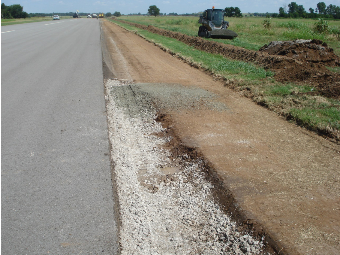
Figure 6.2. Over Excavation Area Filled With Crusher Run Material
