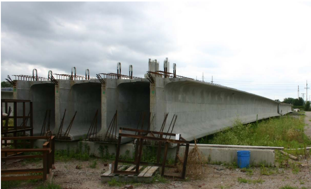
Figure 6.5: Camber in NU-2000 Girders at the Coreslab Plant in Kansas City
