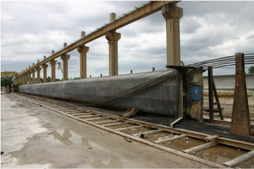
Figure 6.3: Preparation of NU-2000 Form at Coreslab Structures, Inc.
