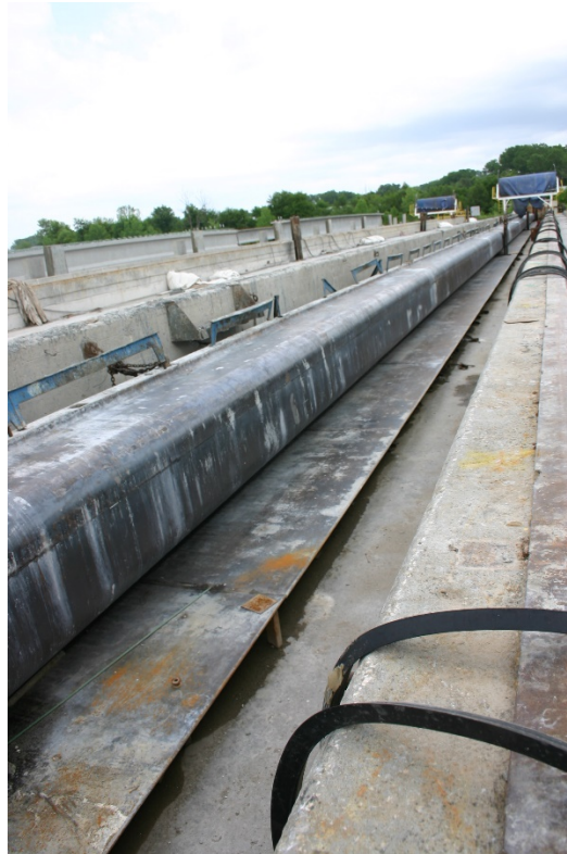
Figure 6.2: Casting Bed with NU-900 Forms at Coreslab Structures, Inc.
