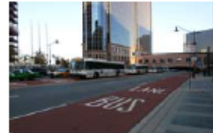
Example of Marking: on Managed Lane
