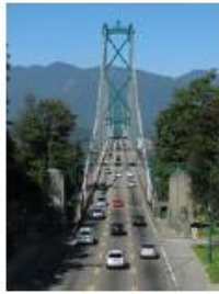
Reversible Managed Lane on Lion Gate Bridge, Stanley Park, Vancouver
