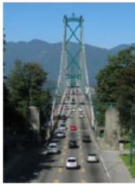
Reversible Managed Lane on Lion's Gate Bridge, Stanley Park, Vancouver
