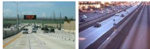
Buffer-Separation in 95 Express, Florida Concrete Barriers in I-15 Express, San Diego
