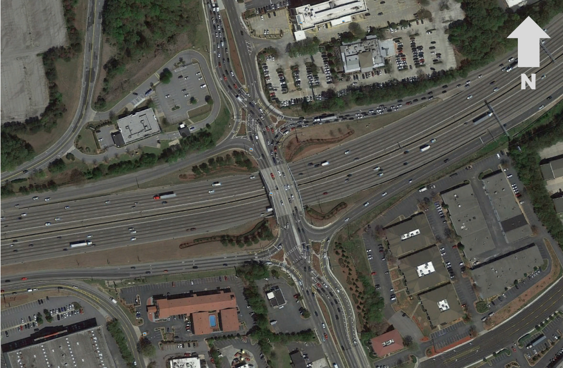
Figure 6: After configuration of the diverging diamond interchange at Jimmy Carter Blvd. and I-85 in Norcross, GA (Google Earth®, accessed 11/28/2017)
