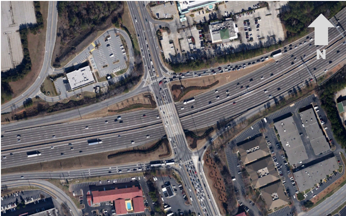
Figure 5: Before configuration of the conventional diamond interchange at Jimmy Carter Blvd. and I-85 in Norcross, GA (Google Earth®, accessed 11/28/2017)
