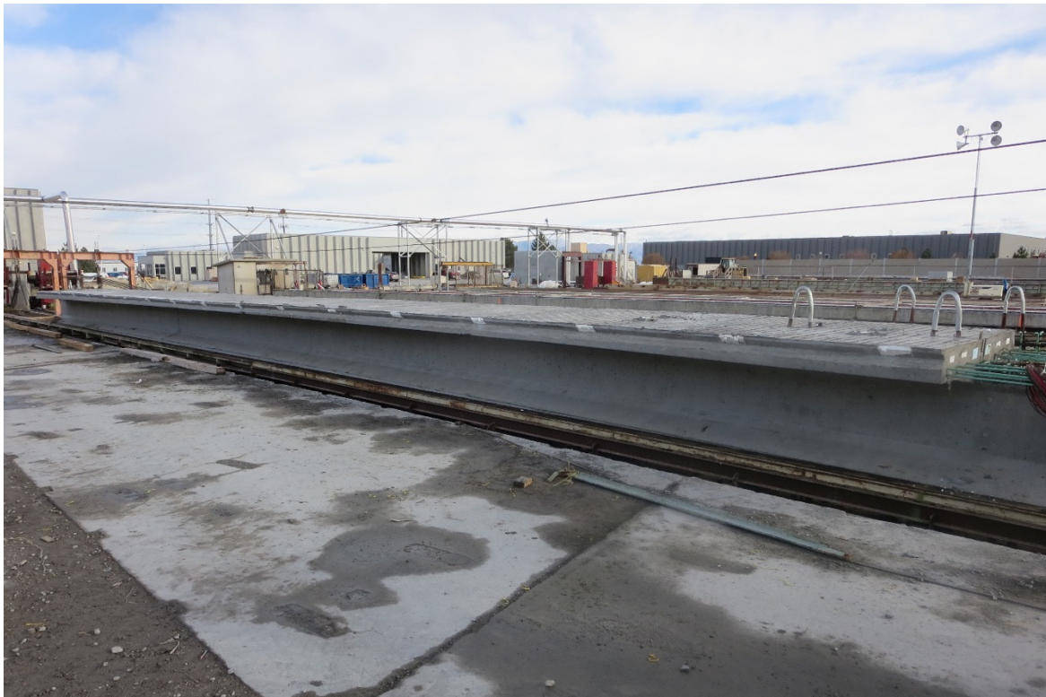
Figure 3.5 Girder in the Casting Bed at the Prestress Yard
