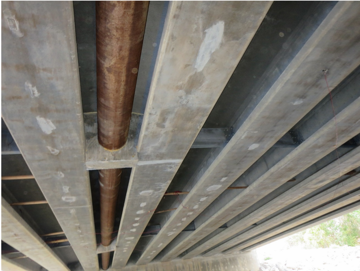
Figure 3.6 Millville Bridge Diaphragm
