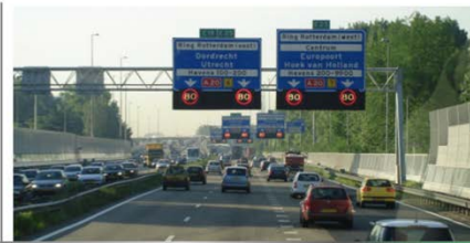
Exhibit 37-5 Variable Speed Limit Signs, Rotterdam, The Netherlands
